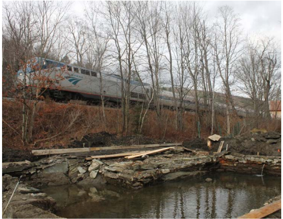
One of Roxbury Fish Culture Stations' rearing ponds that were completely destroyed due to Flint Brook's new water course thanks to Tropical Storm Irene in 2011.
