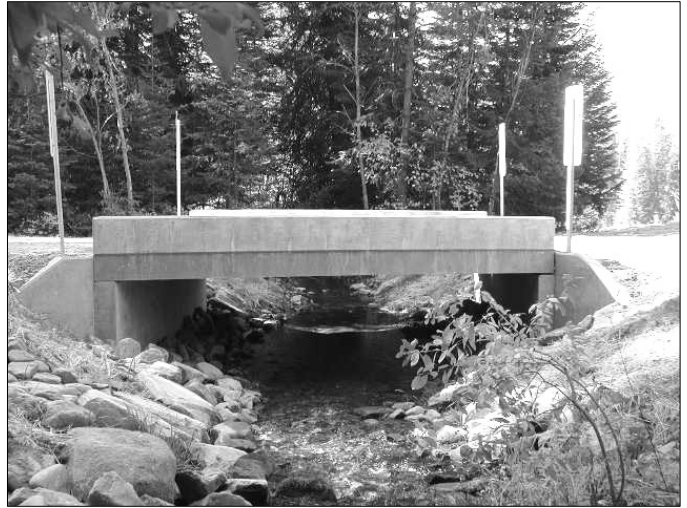
Photo on Left: Culvert failure resulting from water piping. Photo on right: Example of stream simulation construction in bridge
