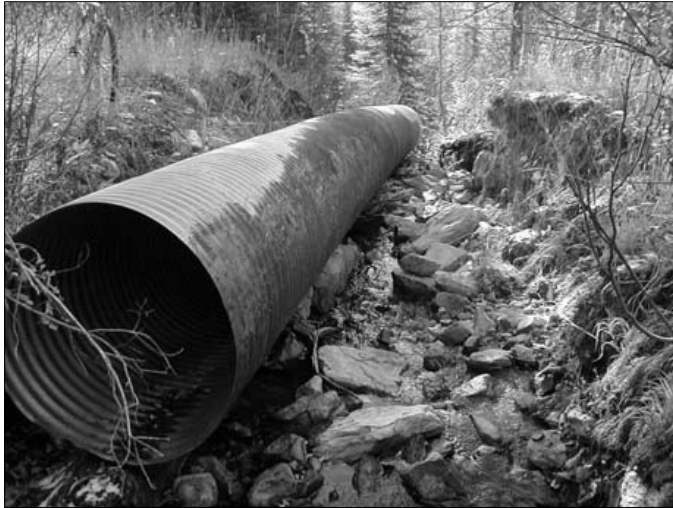
Photo on Left: Culvert failure resulting from water piping. Photo on right: Example of stream simulation construction in bridge
