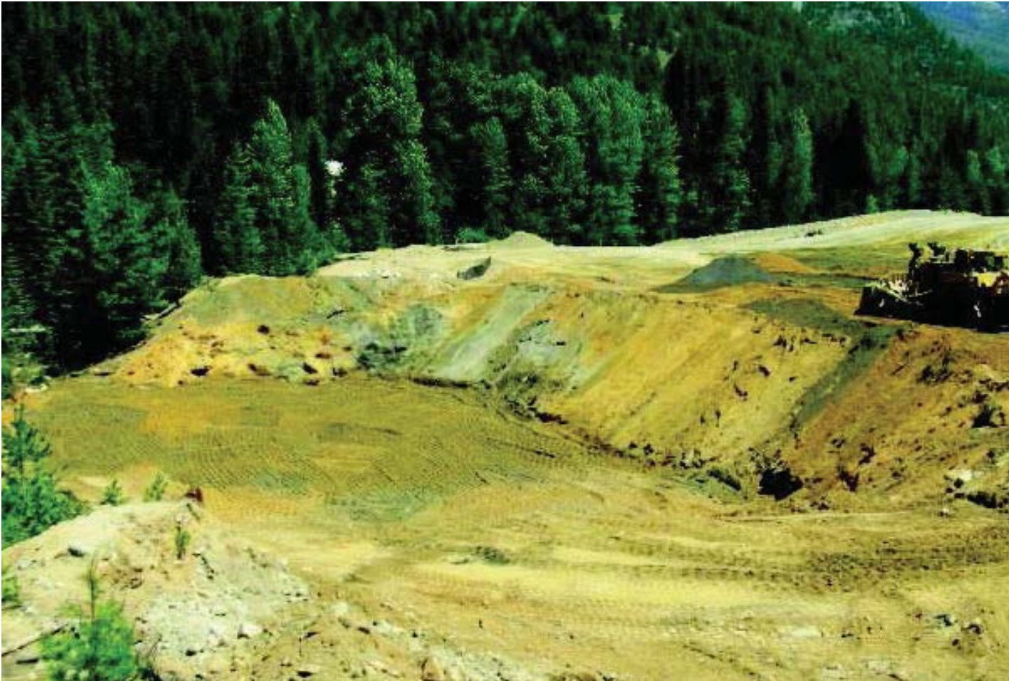
Photos on page 10: Top: Tailings and sawdust placement on east tailings pile 3. Middle: East Copper Creek diversion entering Railroad Creek. Bottom: Compacting the north-west corner of tailings pile 1 following sawdust pile removal.
