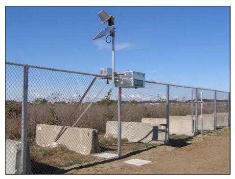
IN DNR has constructed a chain link fence as a barrier to prevent Asian carp from migrating during flood conditions in drainage basins.
