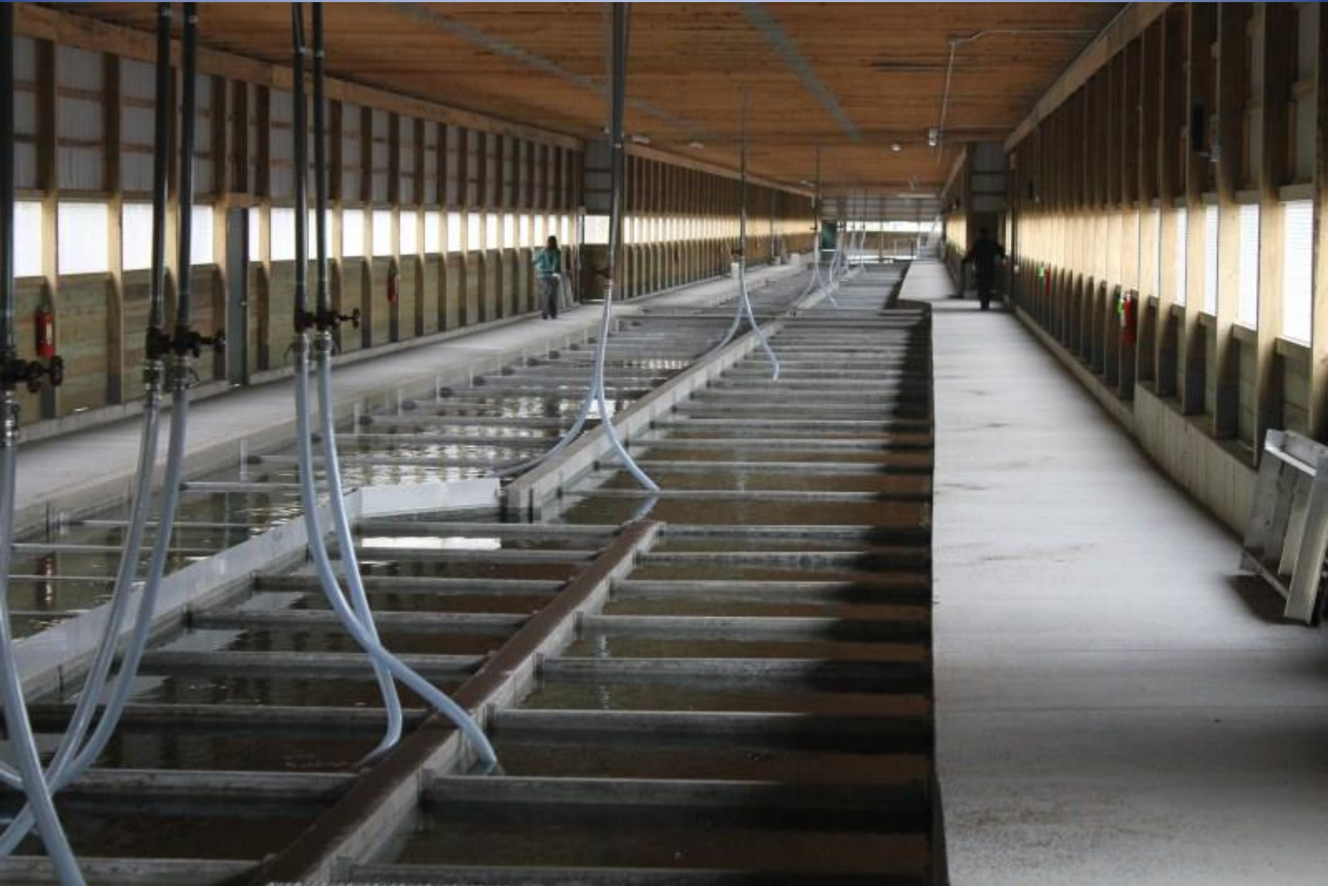
Raceway Enclosure and Aeration system – Production building Water is Reused in Raceways
