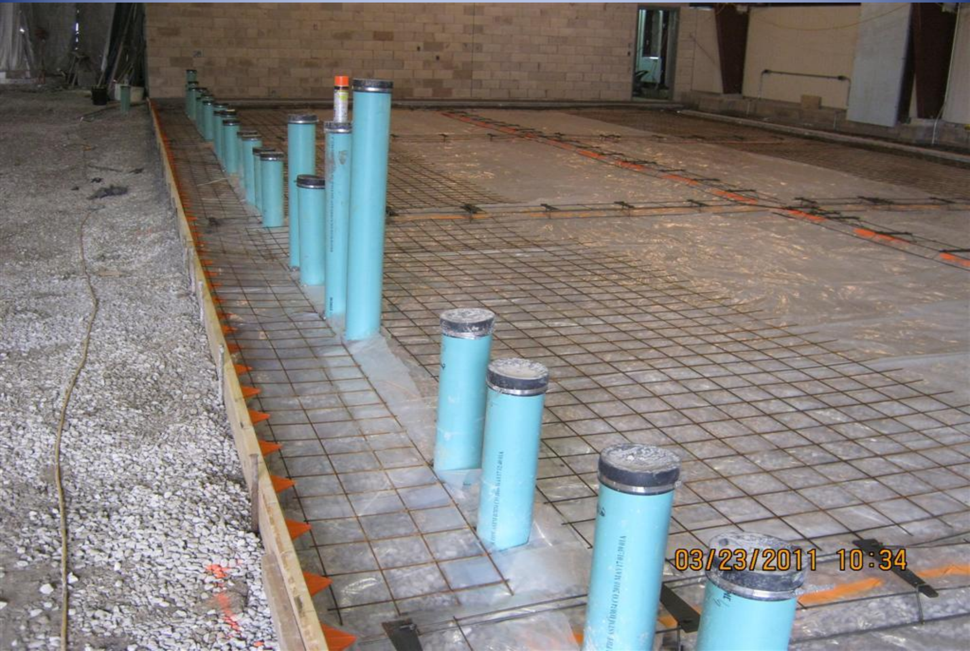
Underground drains installed for the fish rearing tanks.
