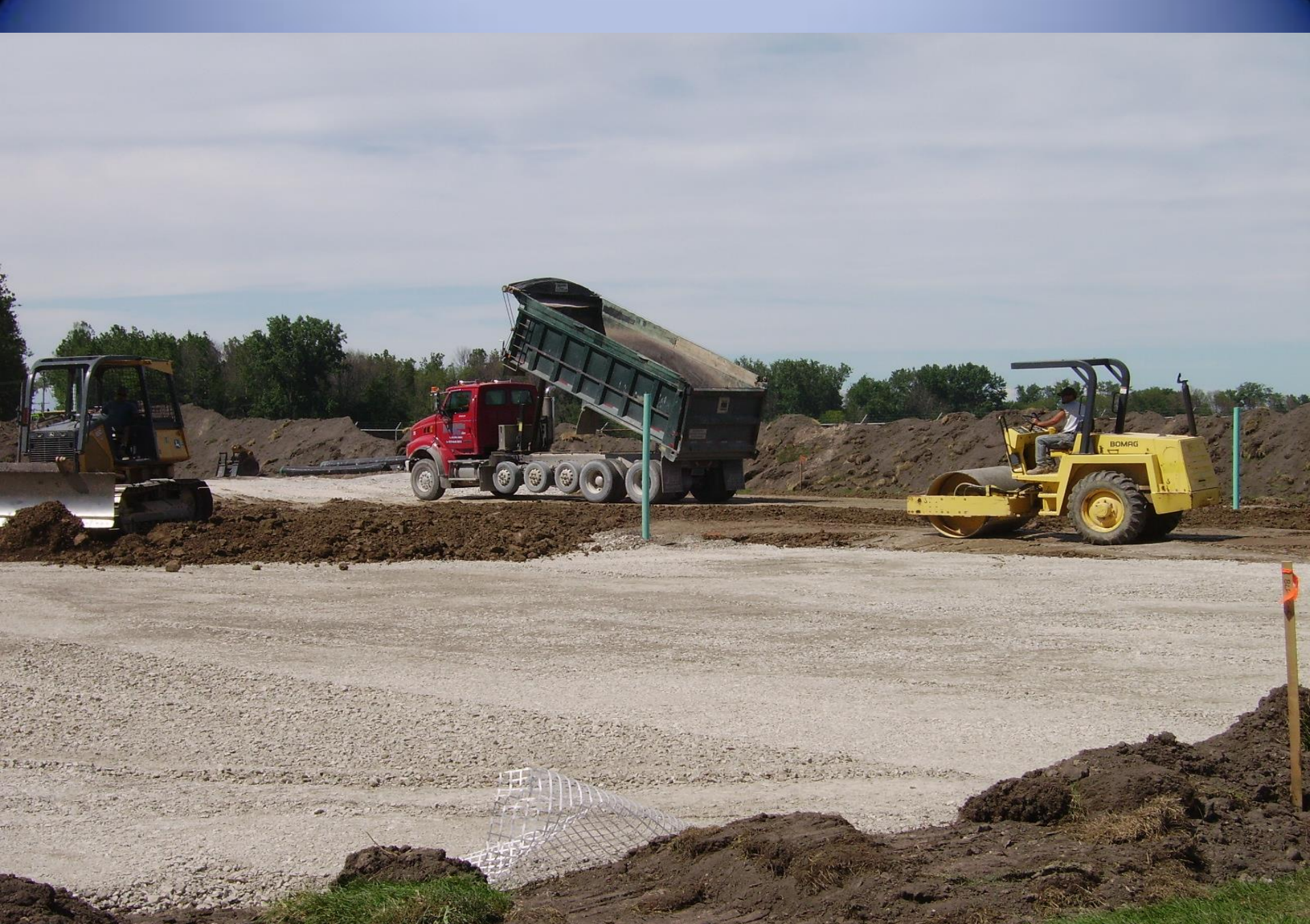
The structural mat is approximately 5 feet thick and has 3 layers.
