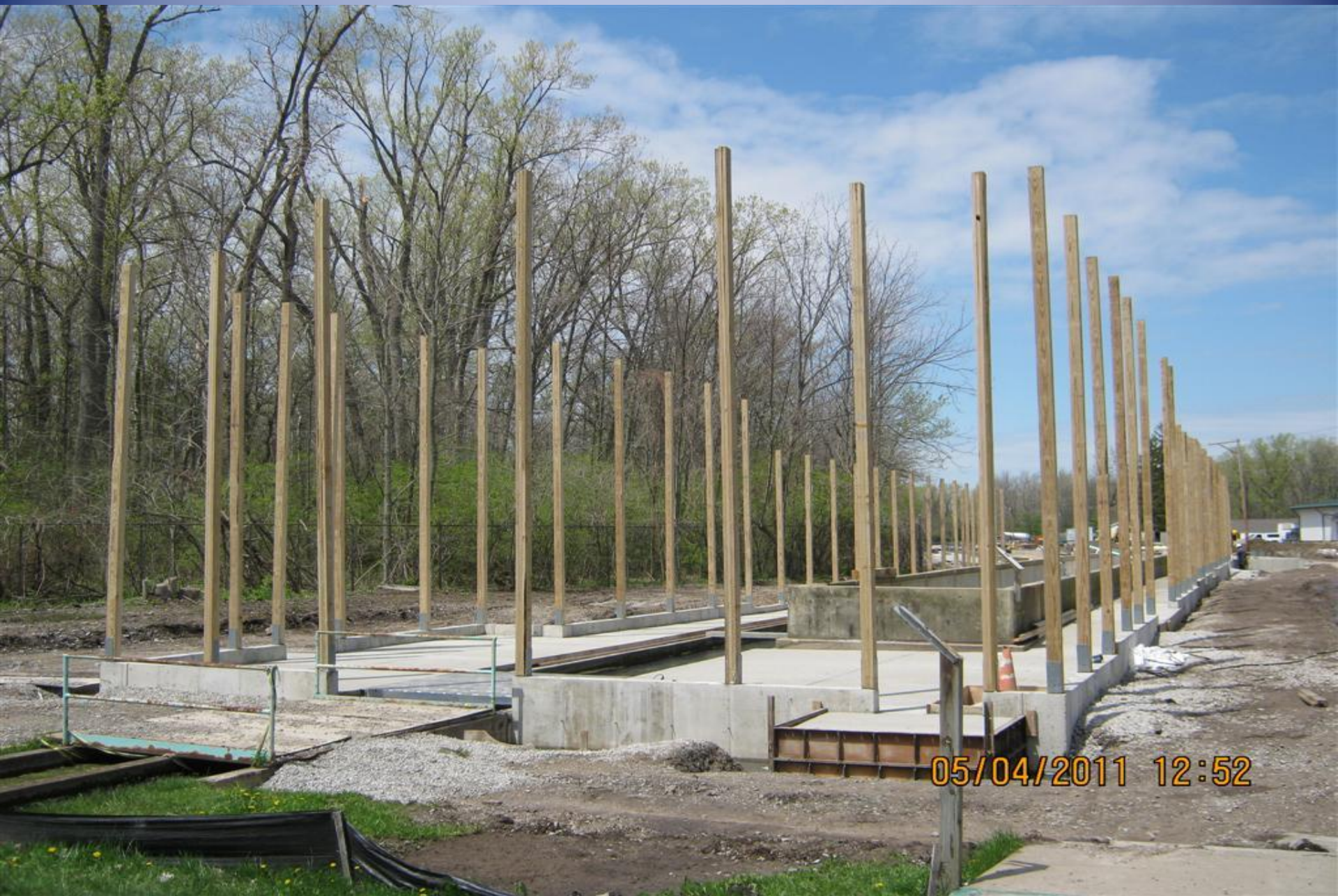
Construction continues on the Raceway Structure.
