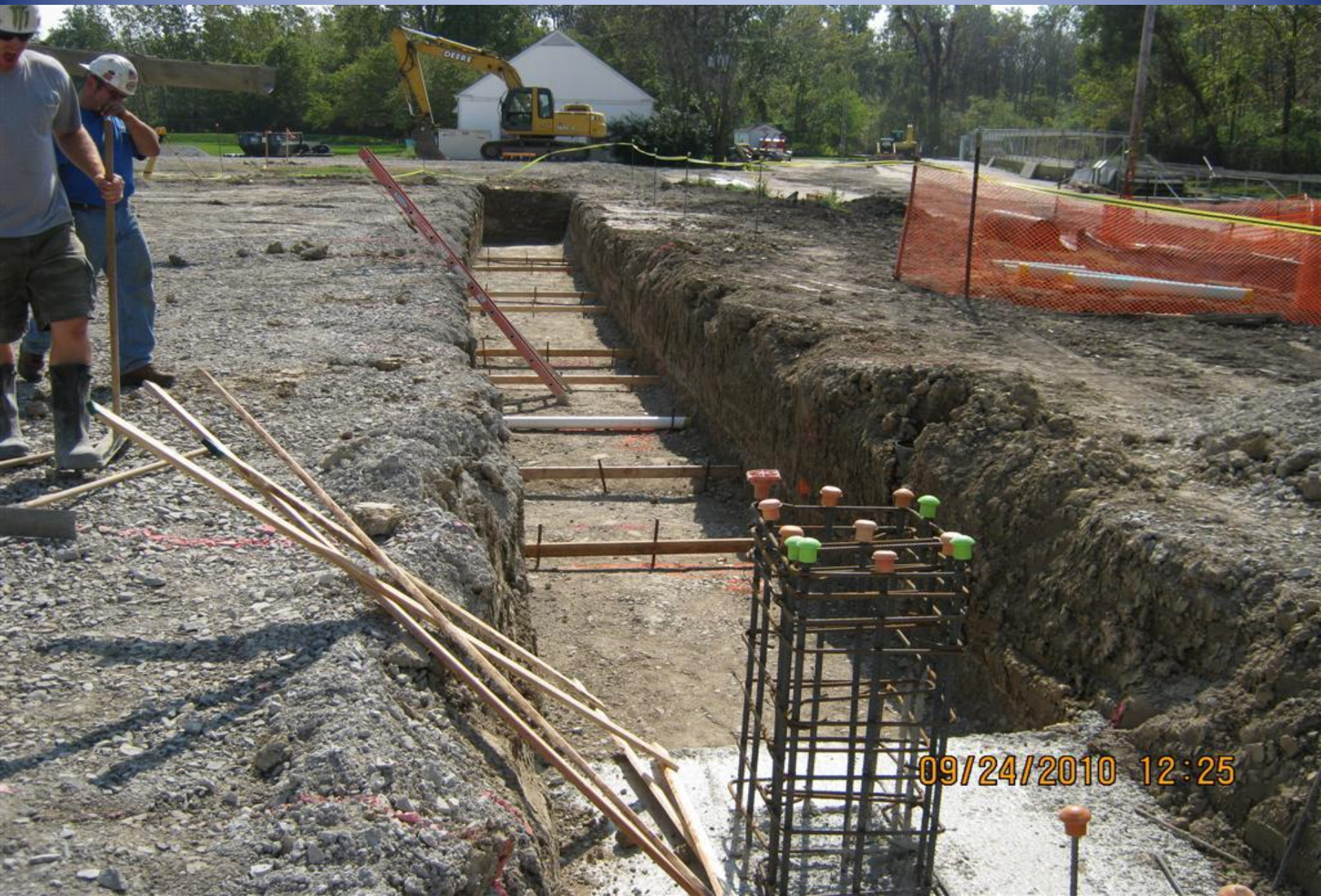
Excavating down to structural mat and start placing foundation.
