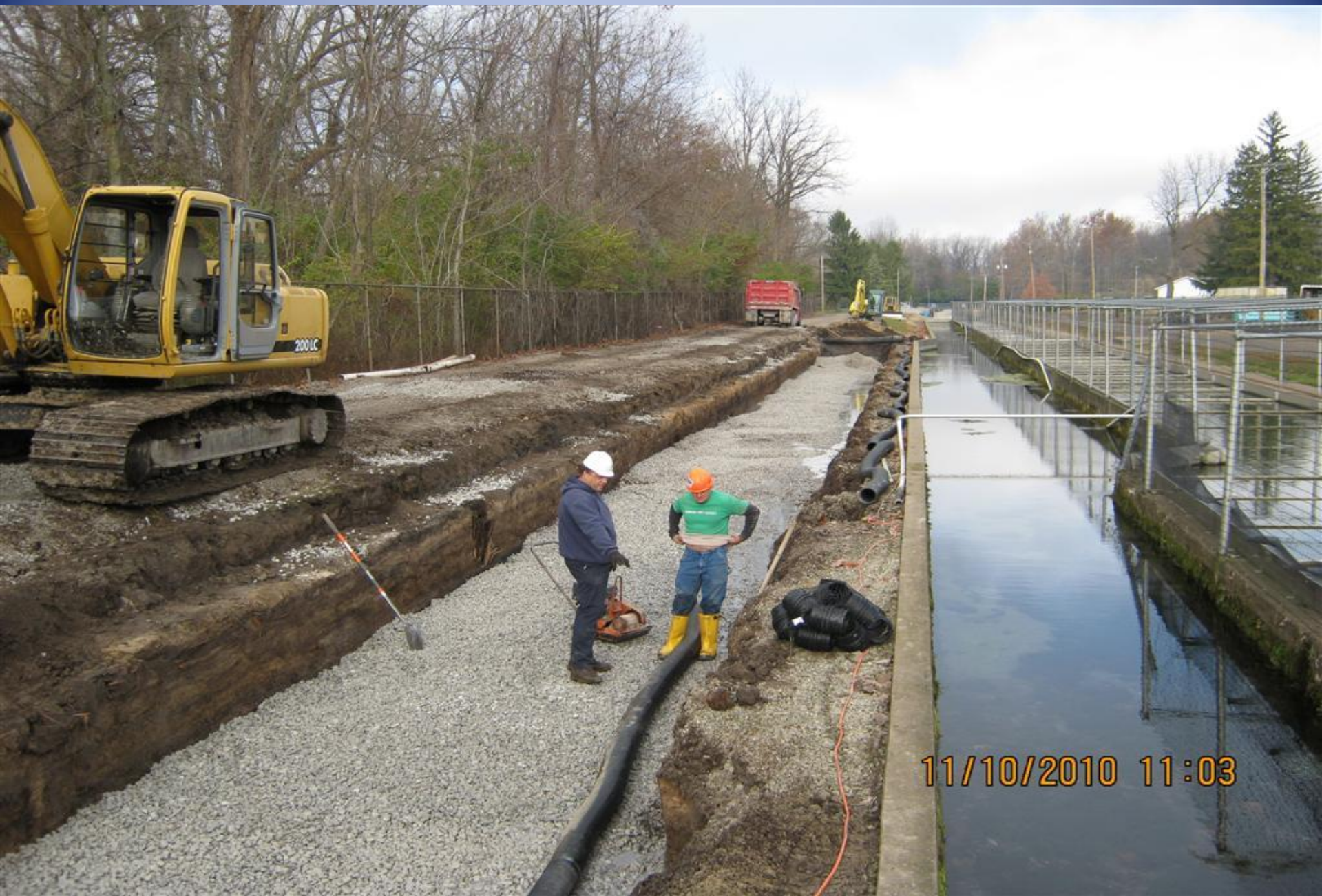
Foundation work on the raceway structure.
