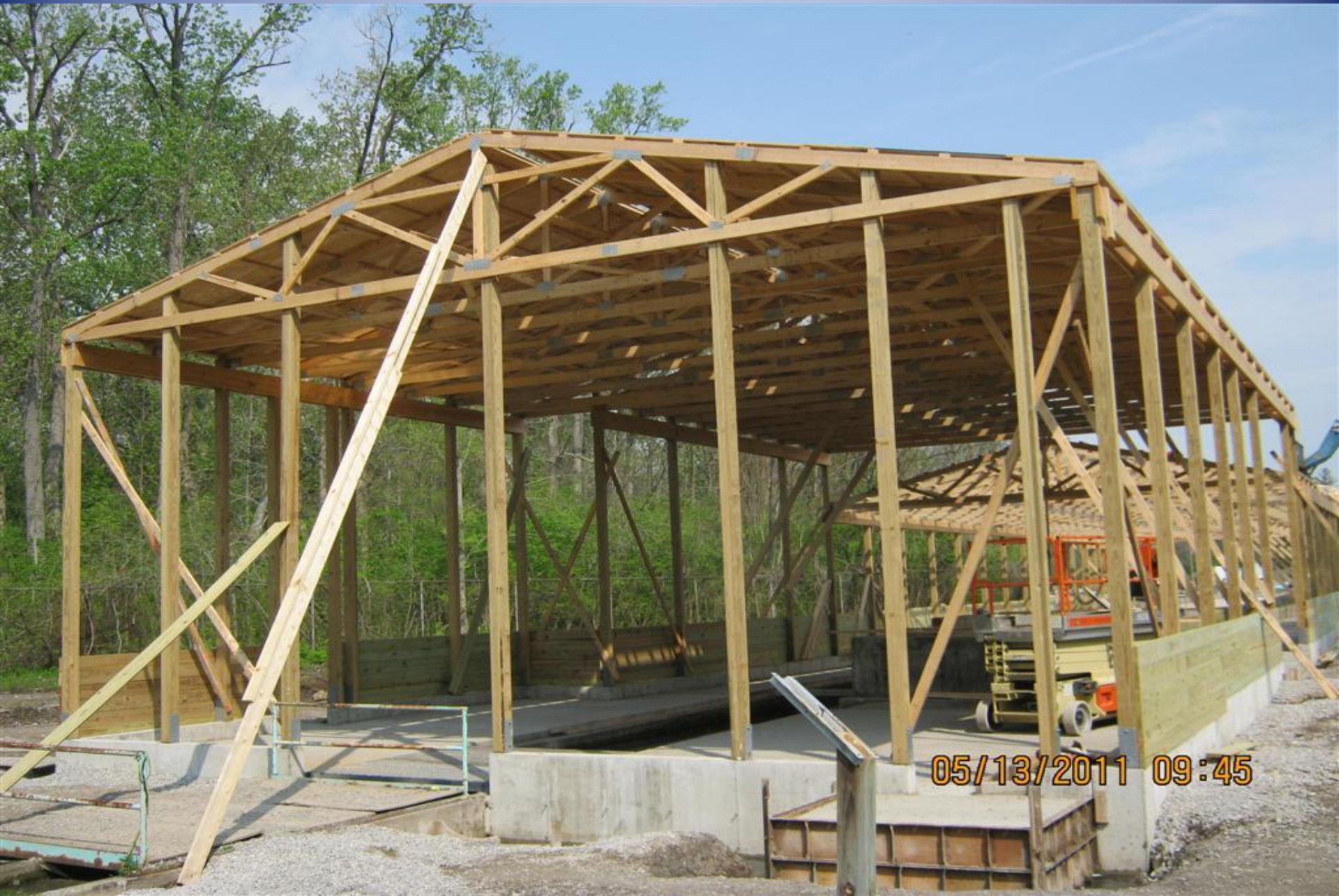
Construction continues on the Raceway Structure.
