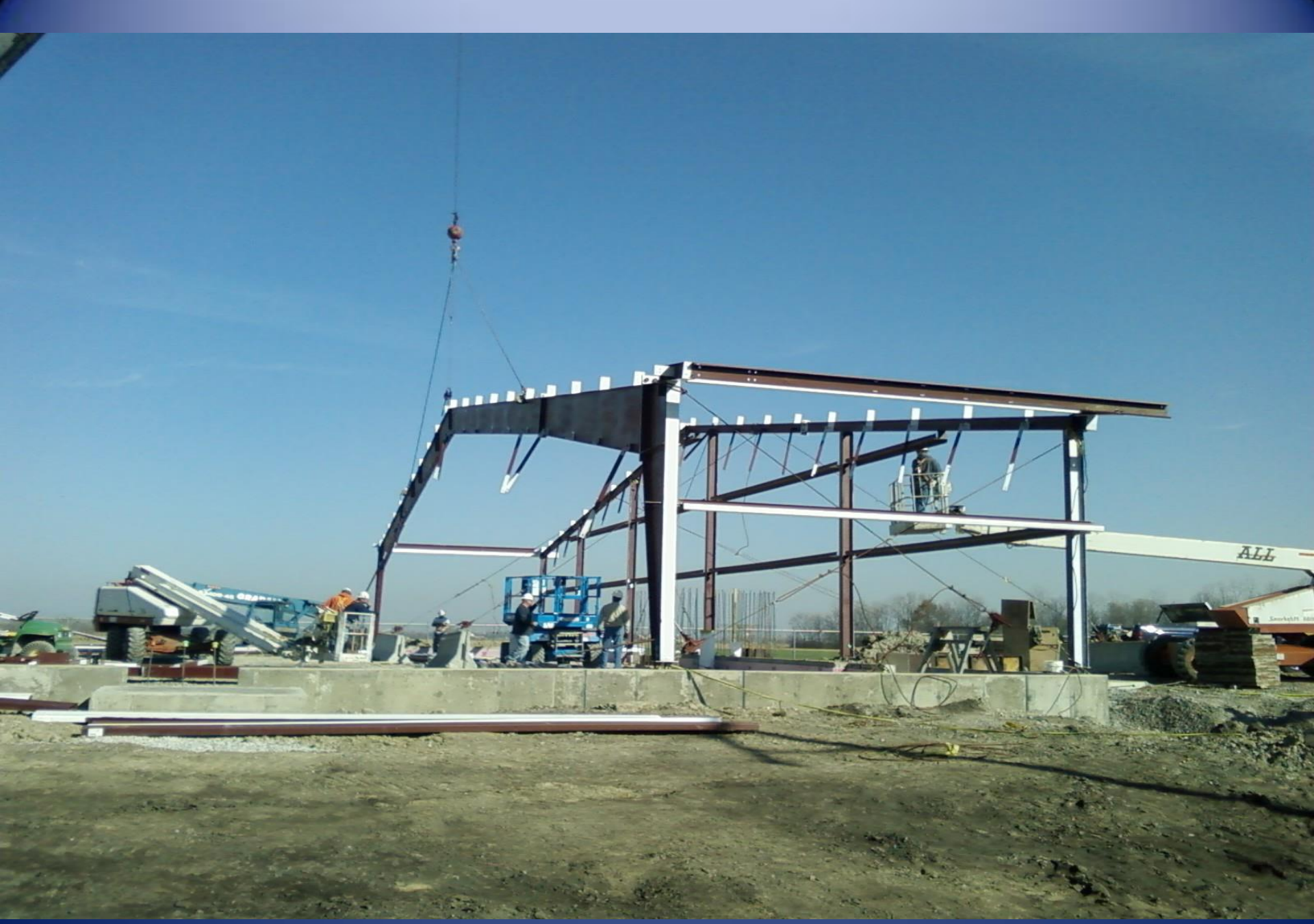
Begin erecting the Hatchery/Production Building
