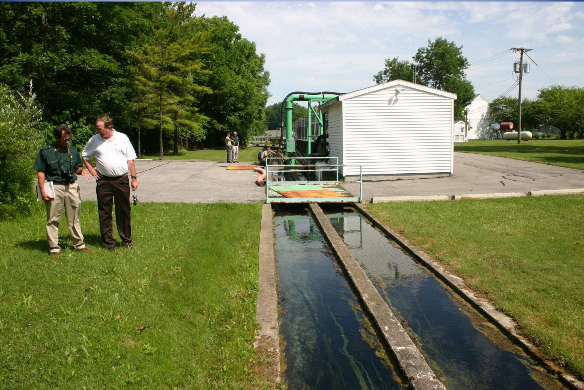
Blue Hole Spring produces 2,500 – 4,000 gpm to original hatchery facility
