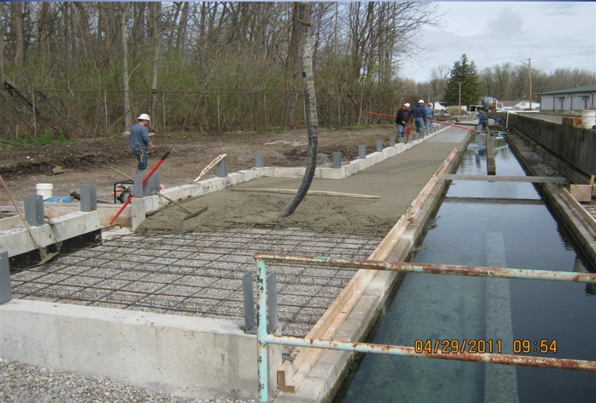
Construction continues on the Raceway Structure.
