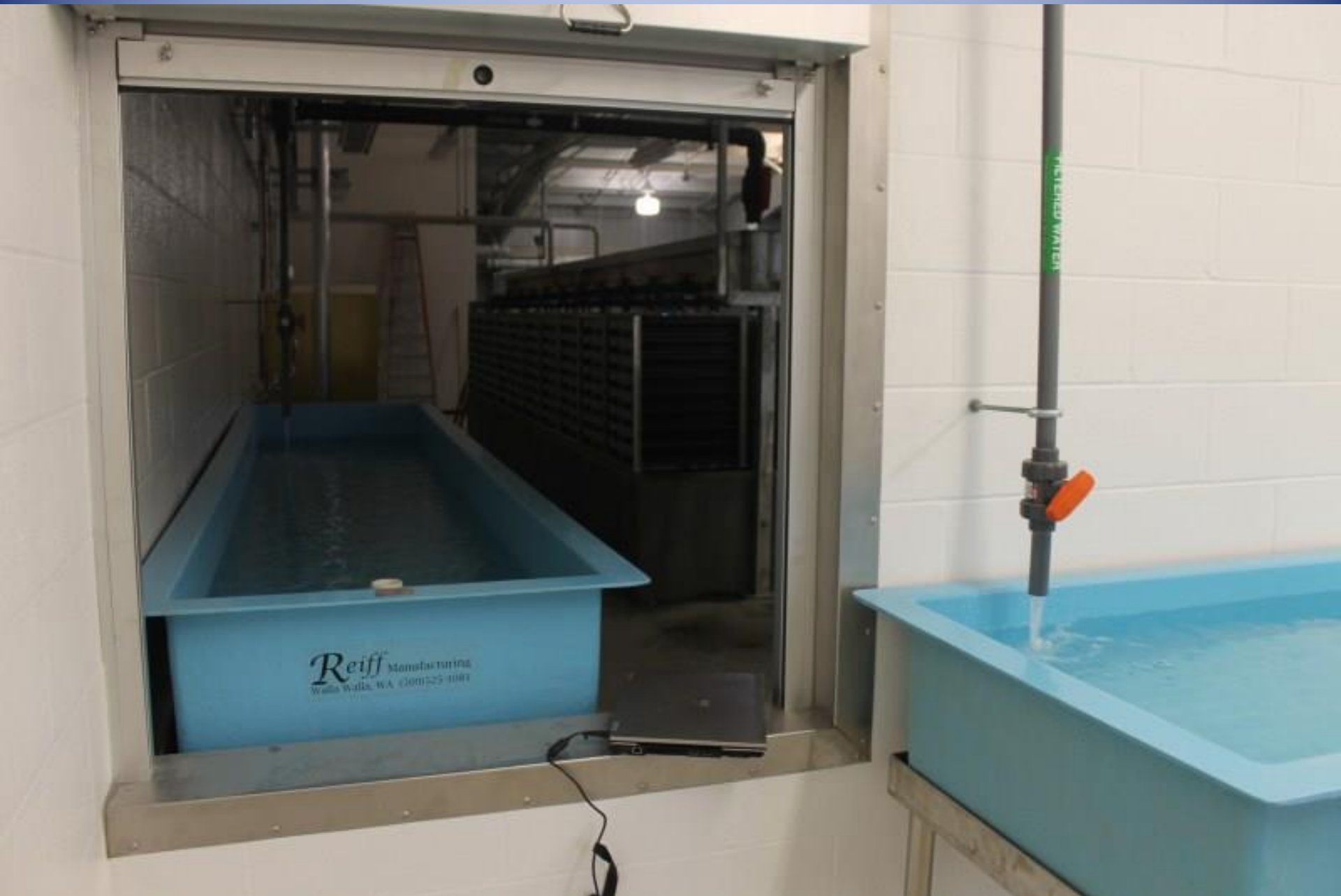
Biosecure Egg Disinfection Room – Egg Washing Troughs & Pass through Window to Incubation Area
