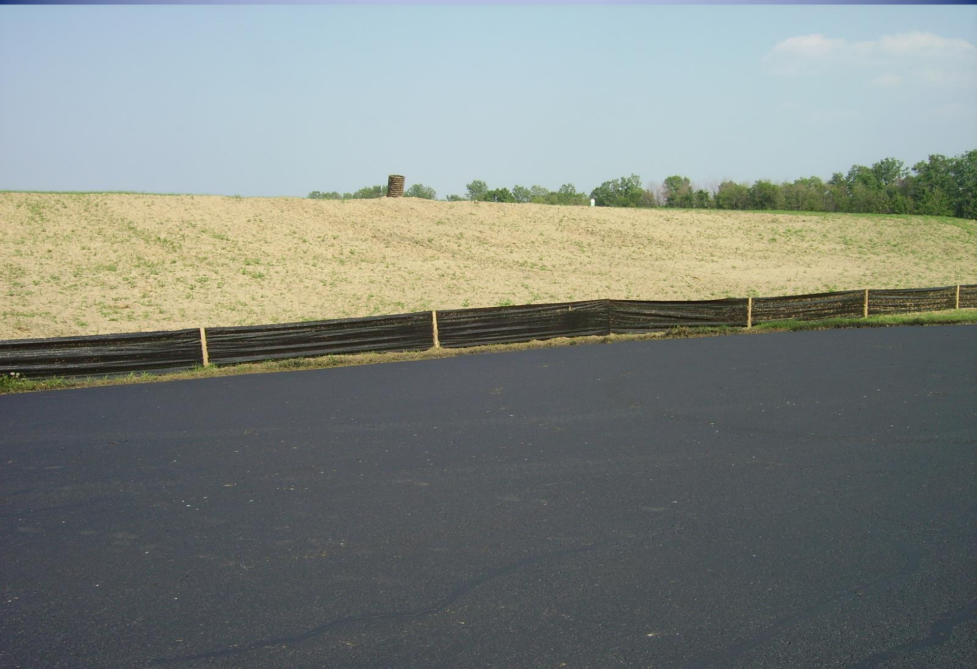
Structural mat and overburden rises 8 ft above the original grade.
