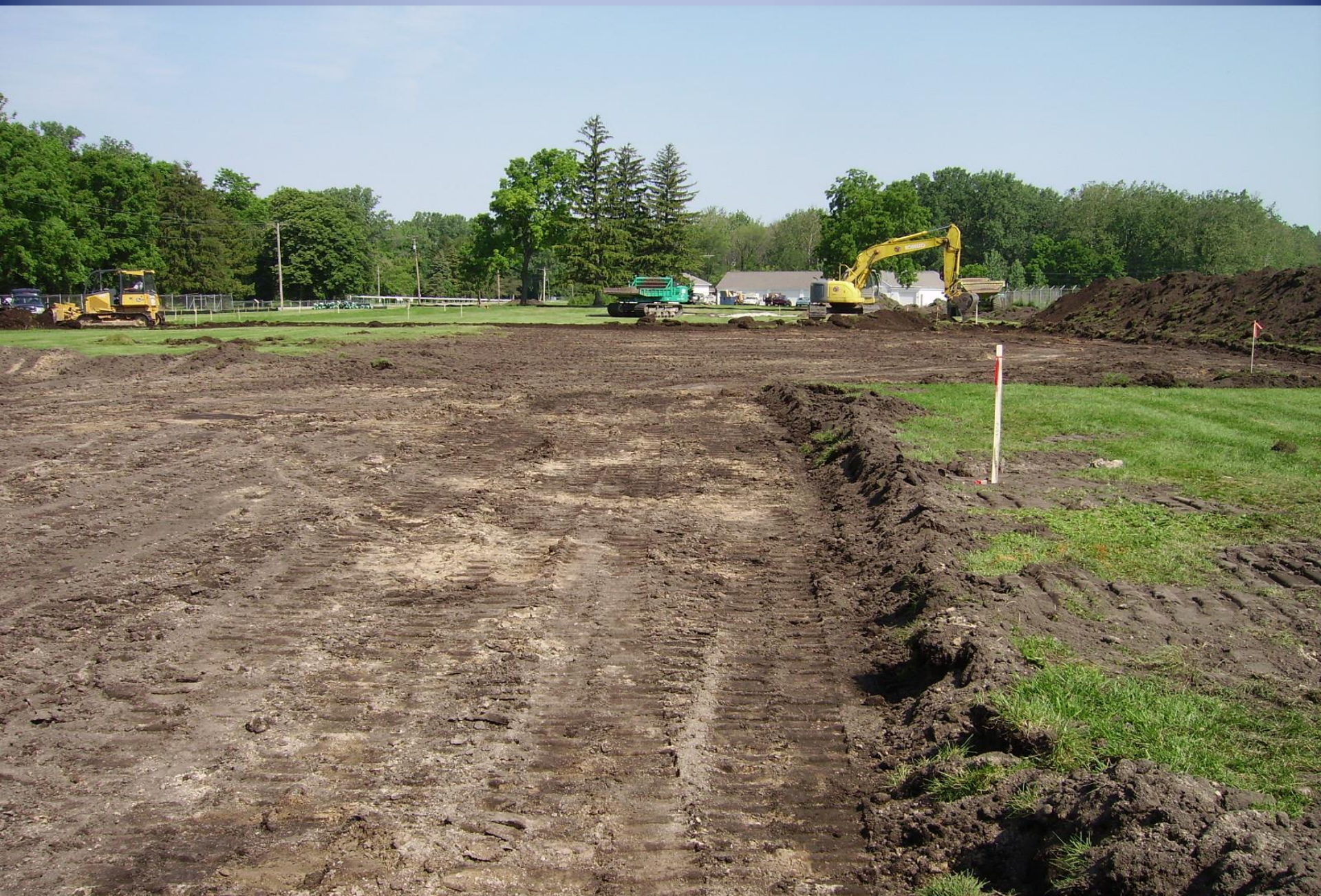
Removal of organic soil for production building construction site.
