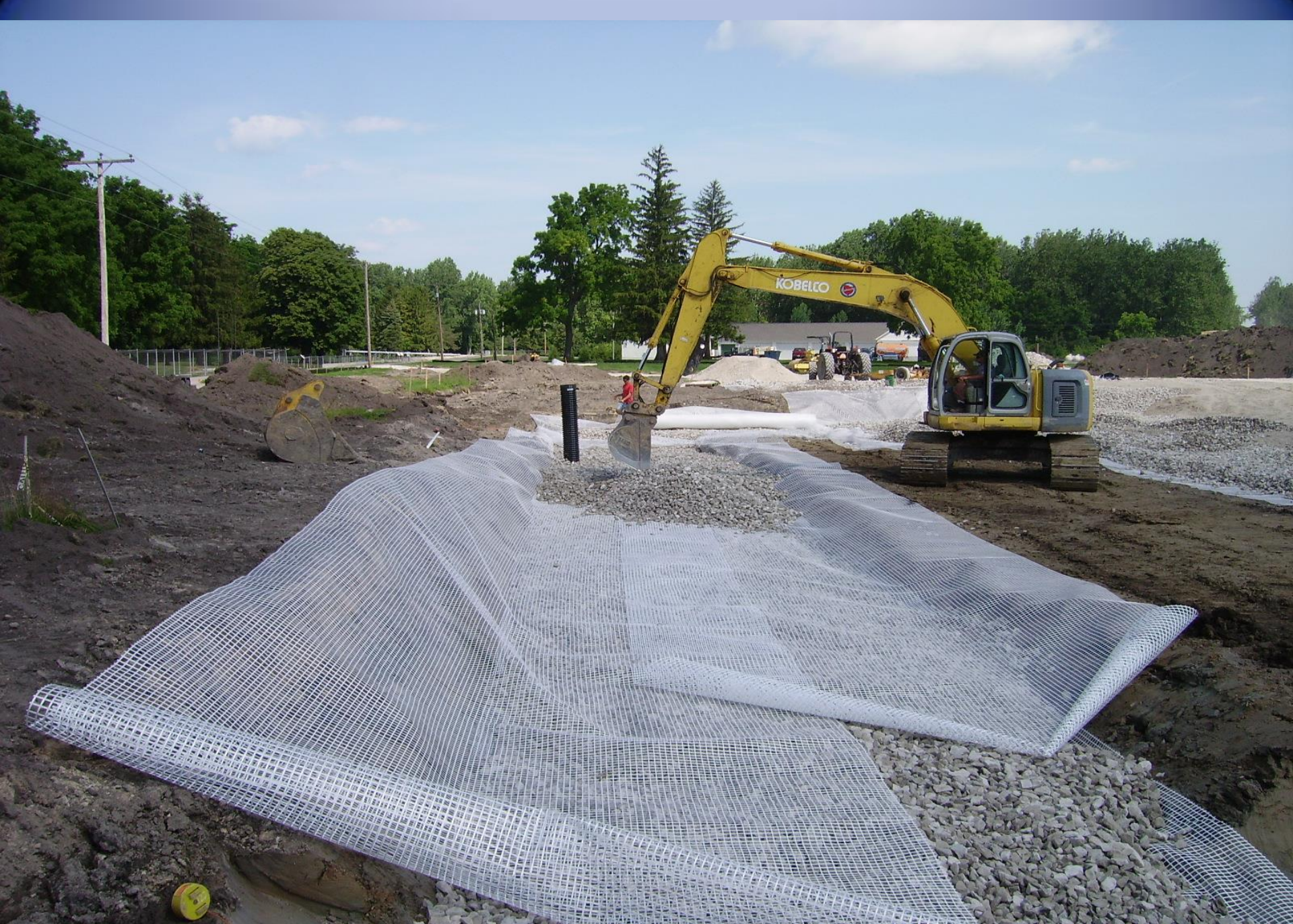
Placement of geogrid and aggregate structural mats (3 layers)
