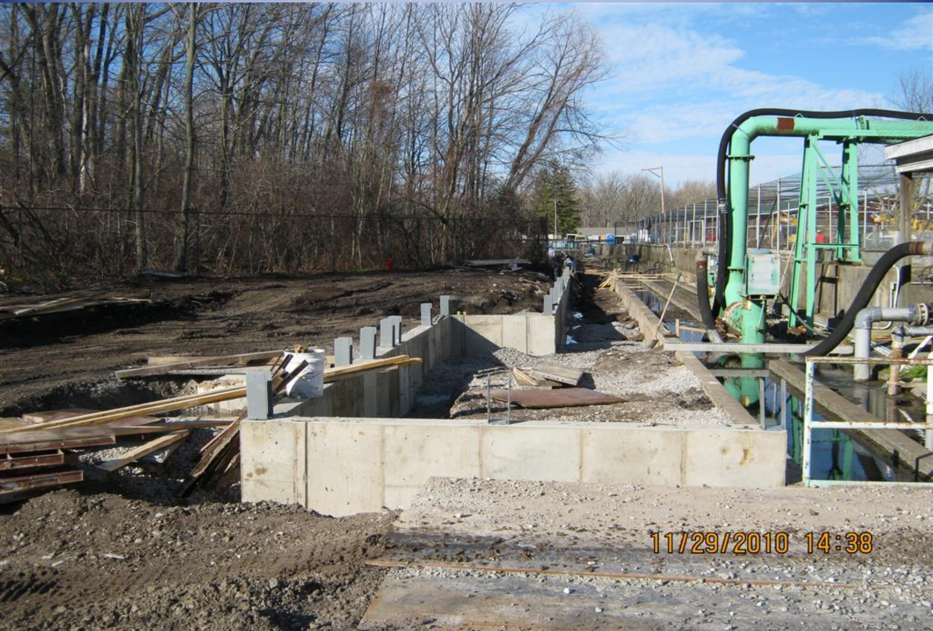
Foundation walls poured on the raceway structure.
