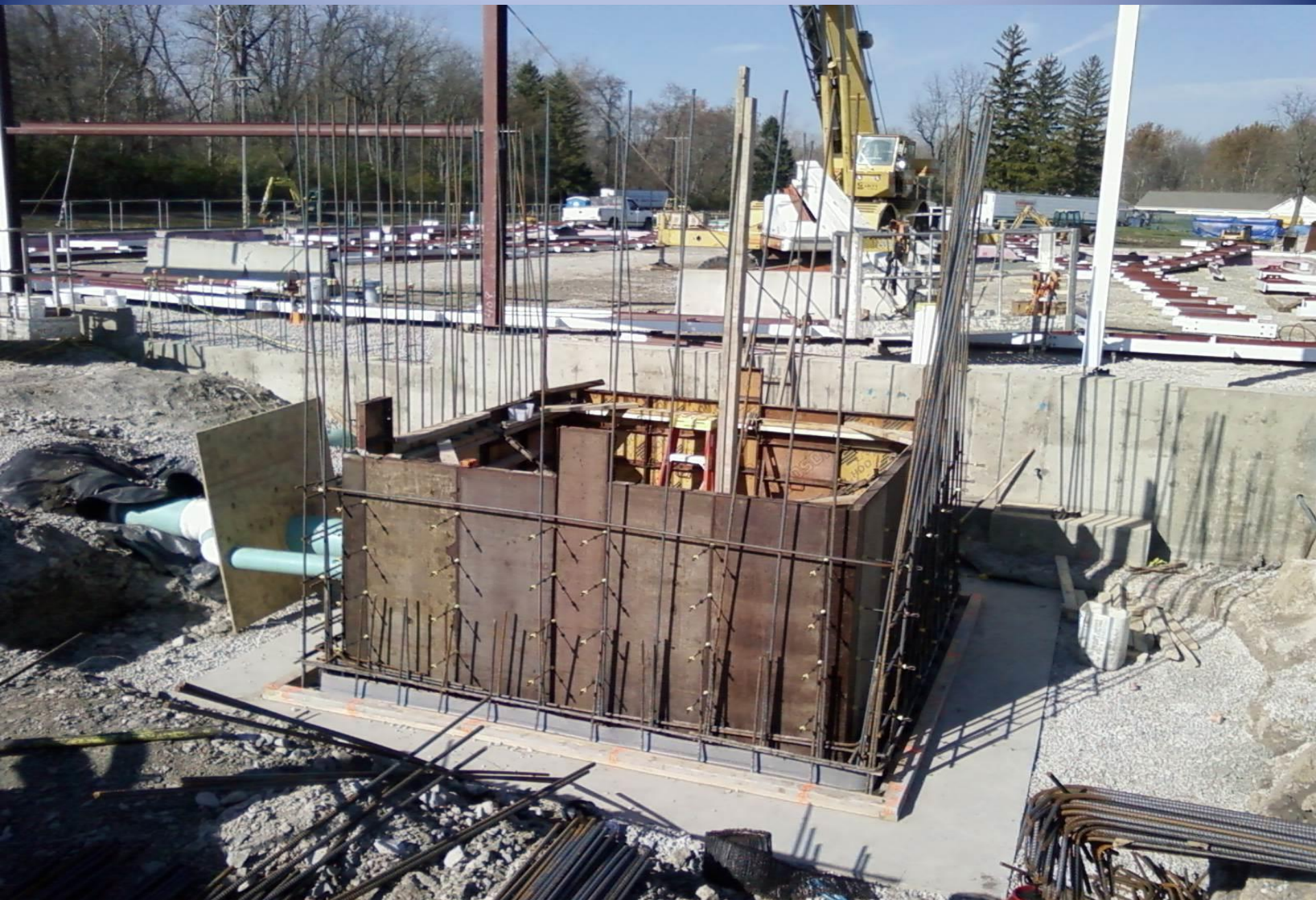
Begin constructing the water supply headtank at the production building
