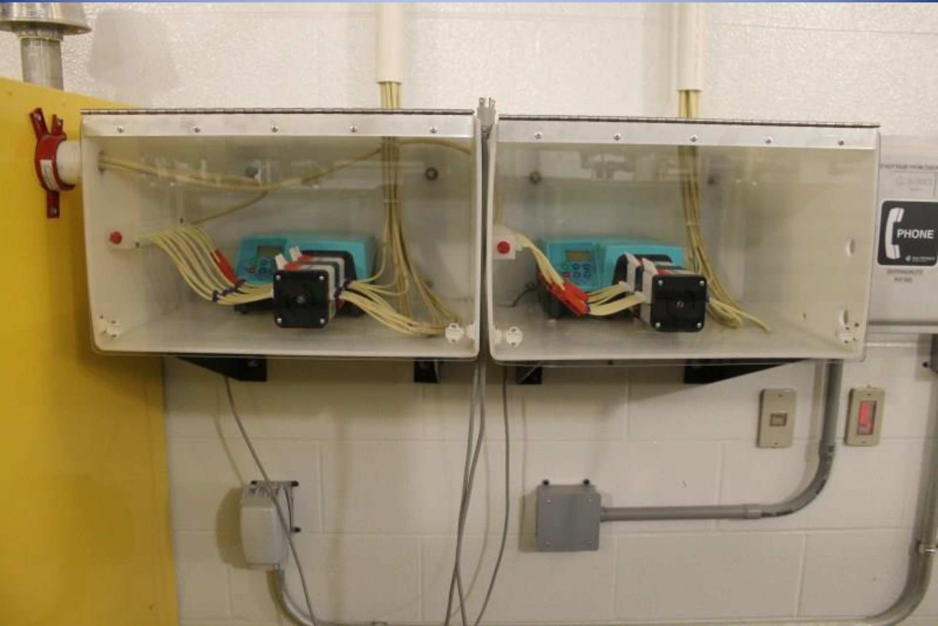
Incubation Area --Egg Fungus Control Metering Pumps
