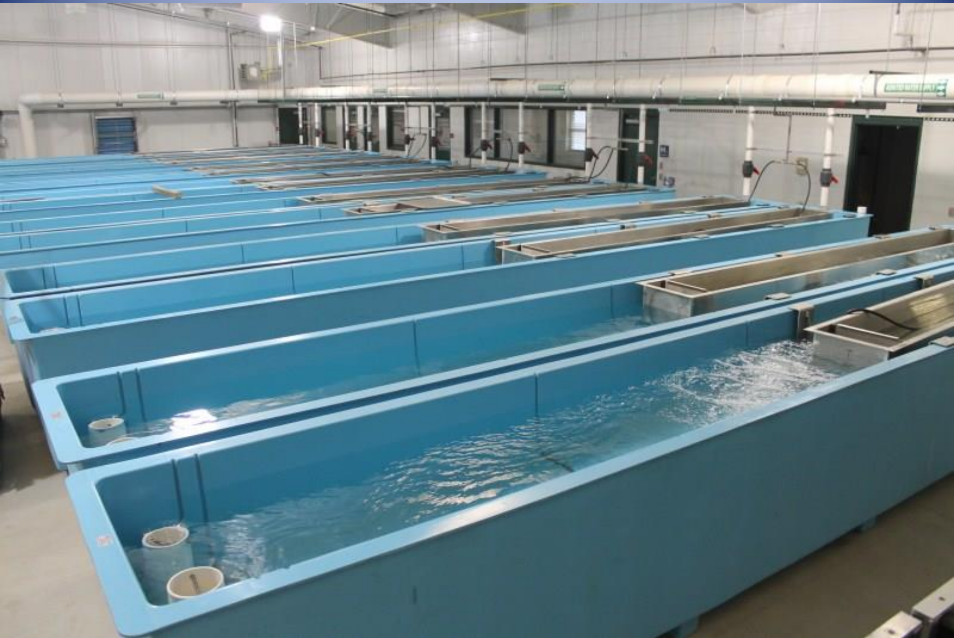
28 – 30 ft x 3 ft x 3 ft FRP Tanks with Portable Aluminum Initial Feed Training Troughs
