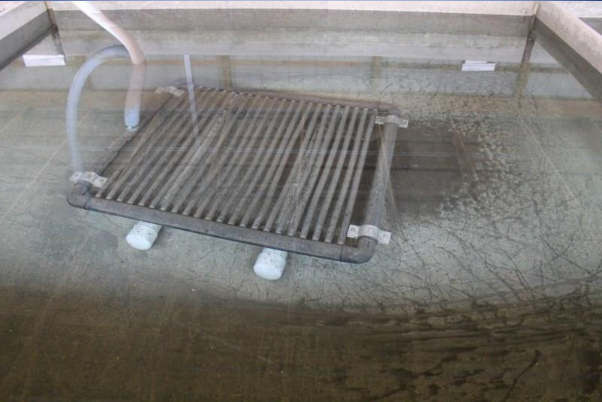
Removable Colorite Aeration Tubing Aeration Sled in Raceway
