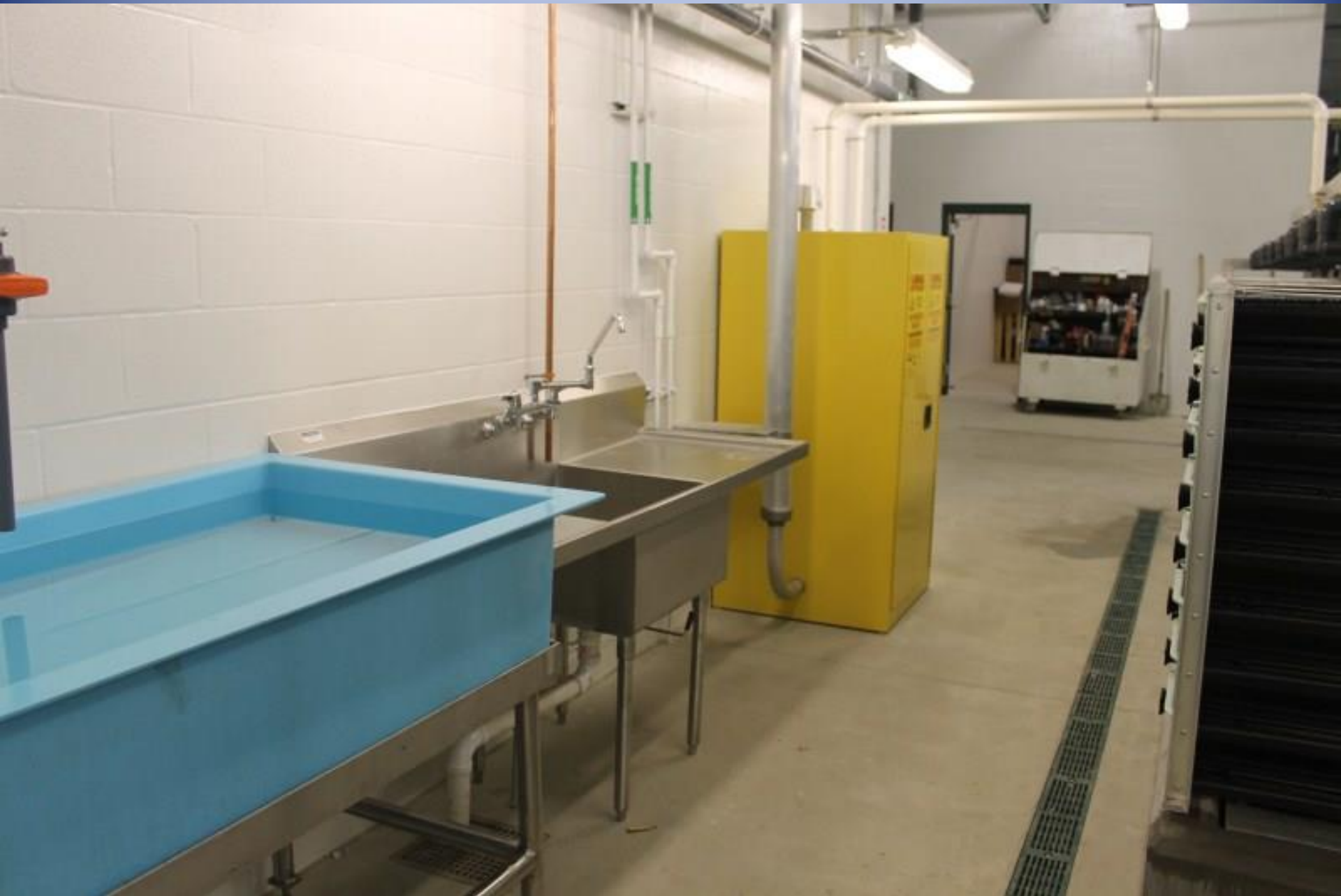
Formalin / Hydrogen Peroxide Vented Chemical Storage in Incubation Area
