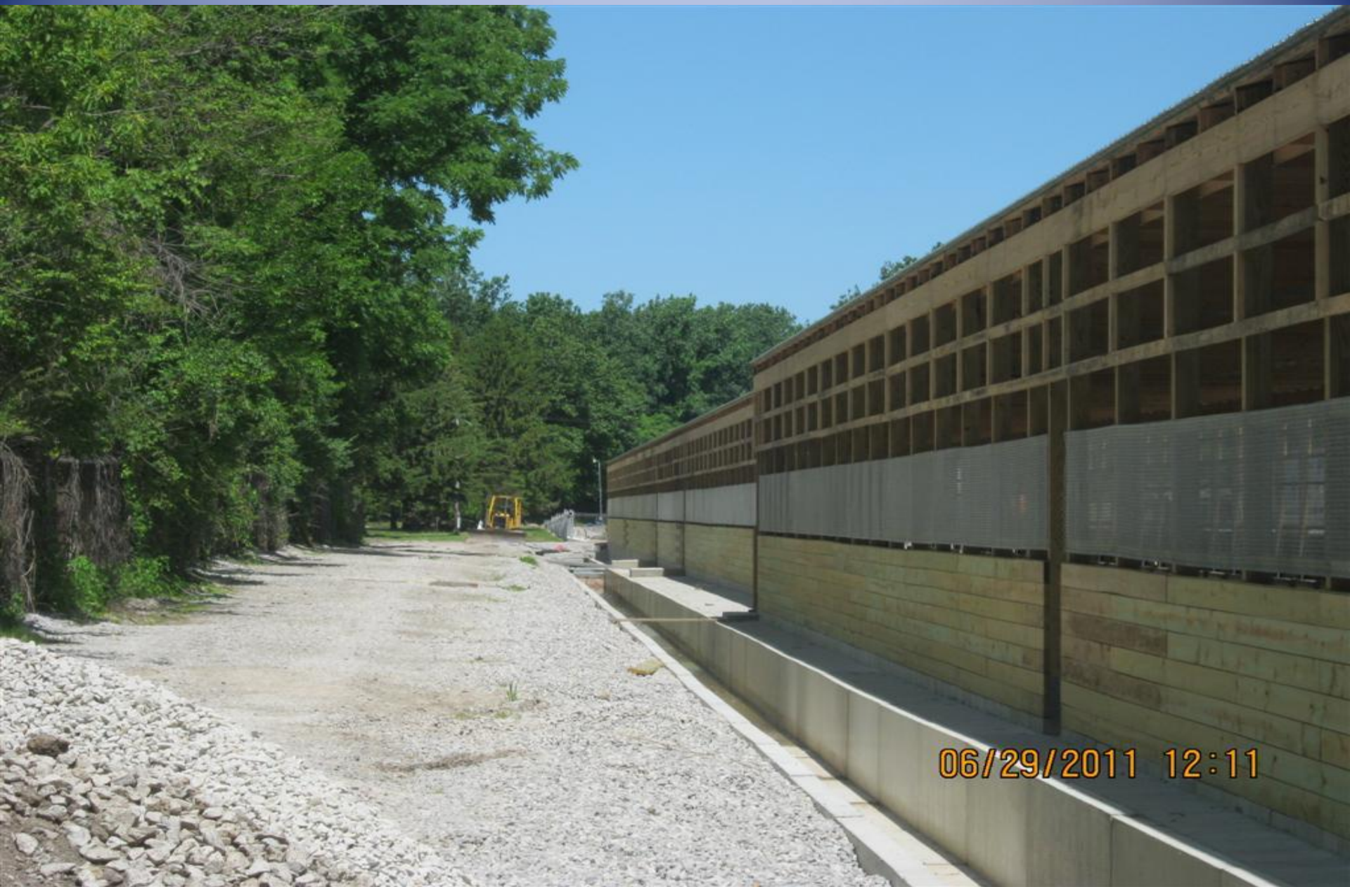
Raceway Structure and by-pass channel almost complete.
