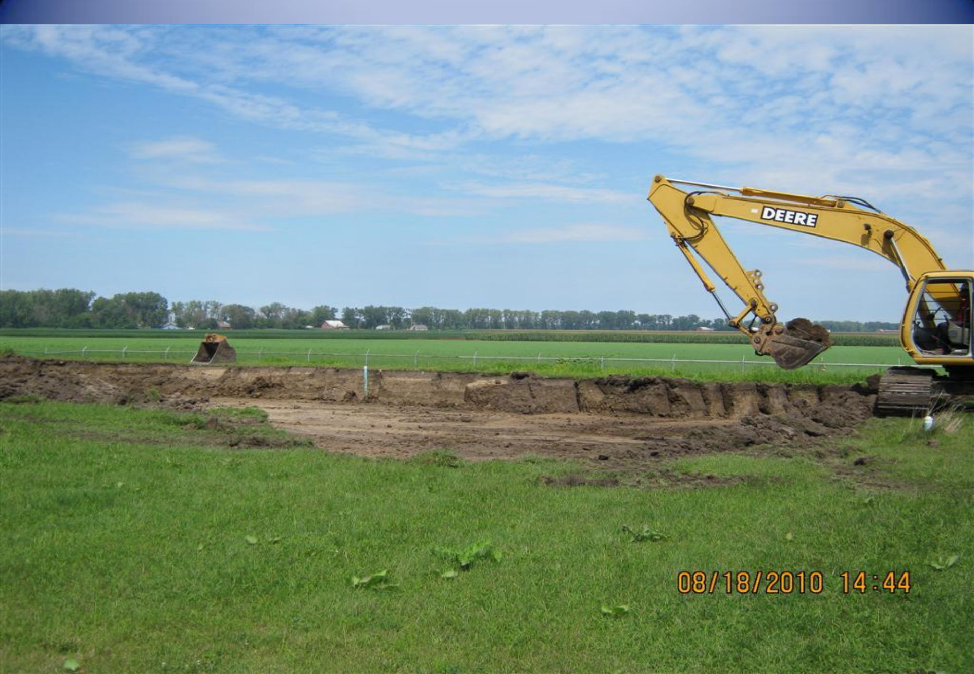
Contractor starts by removing the top 4 feet of overburden.
