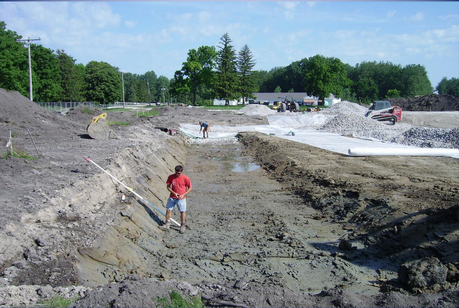
Removal of four (4) feet of original earthen material.
