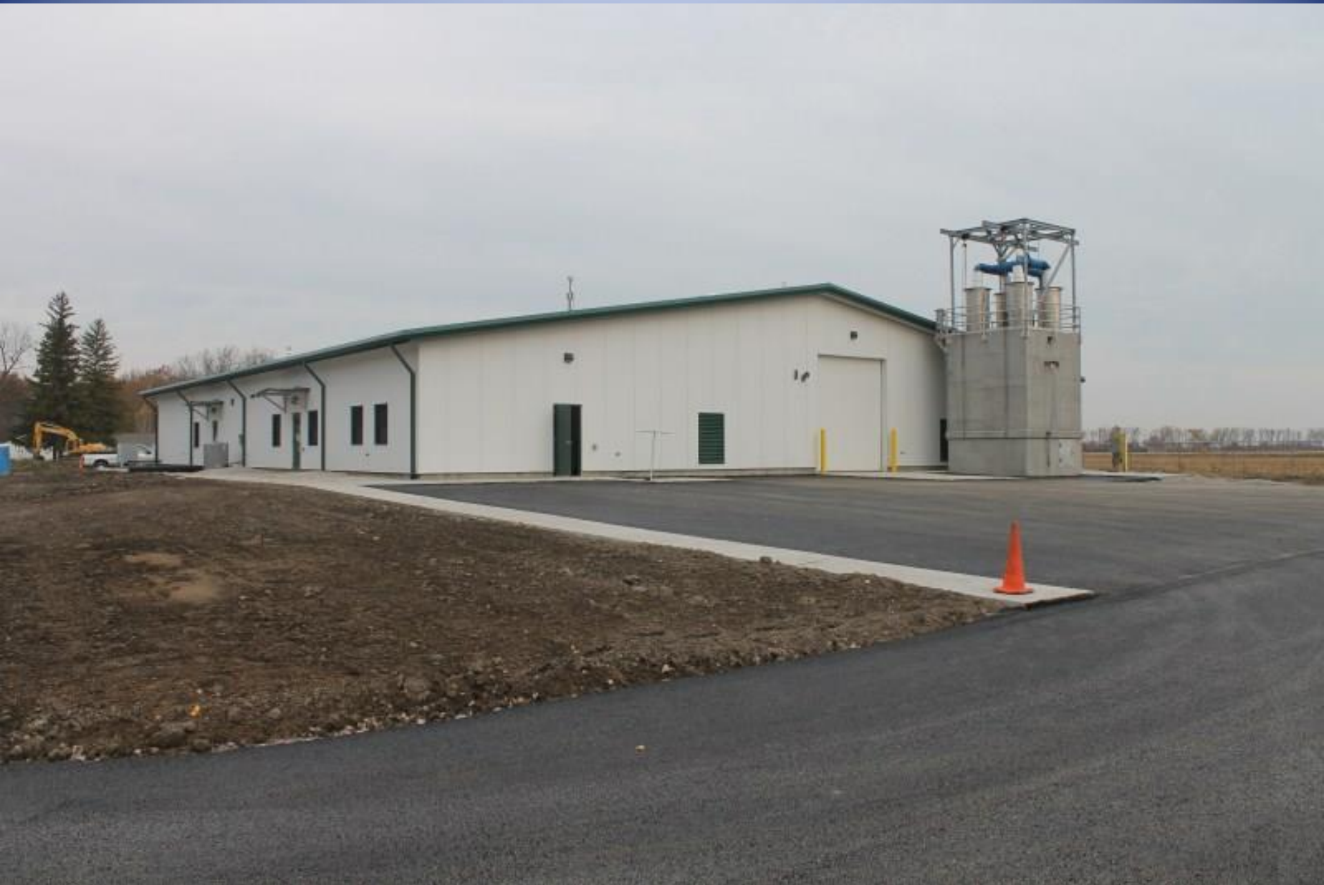
New Production Building & Water Supply Headtank
