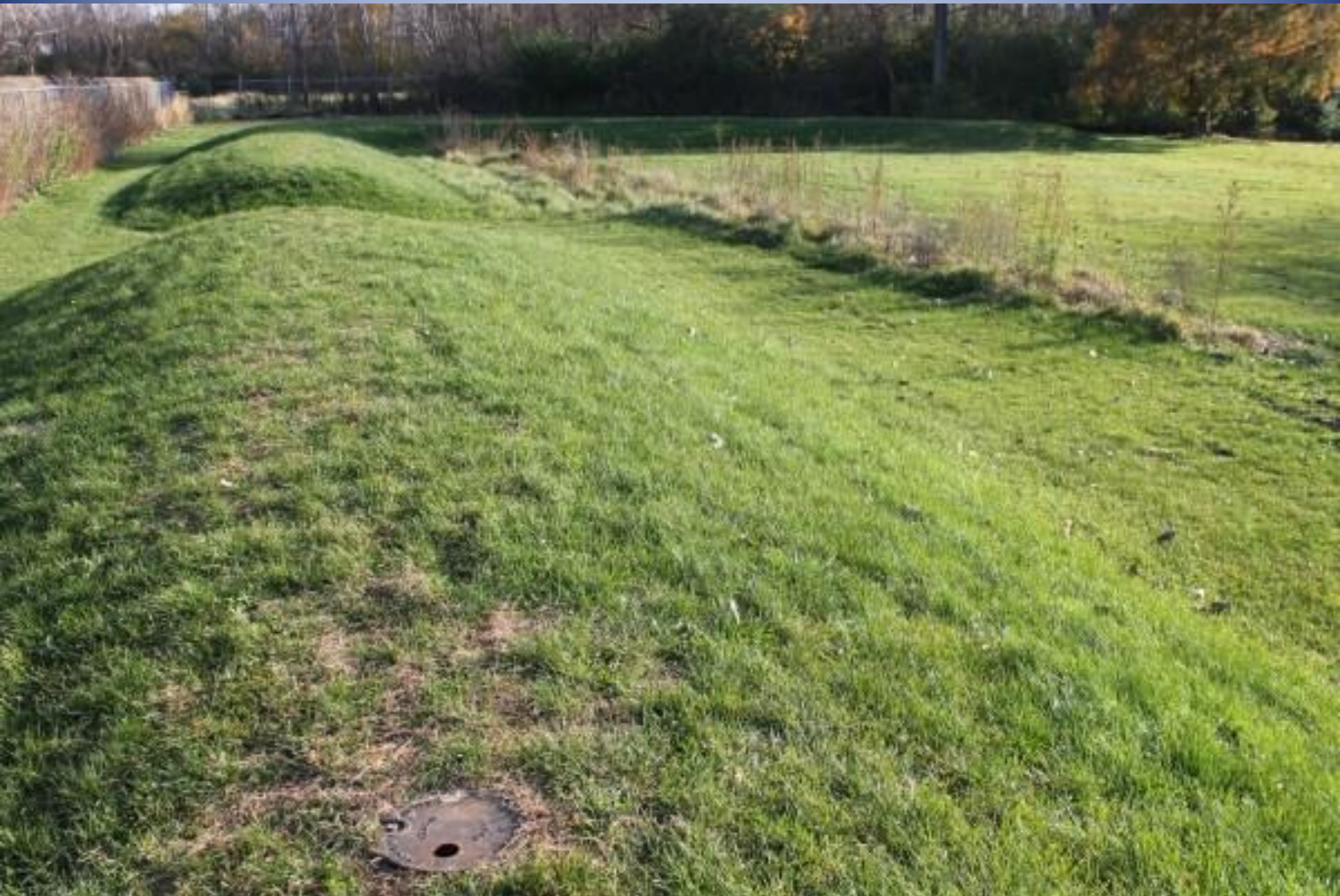
Above grade domestic wastewater leach fields – one used now and one for future use
