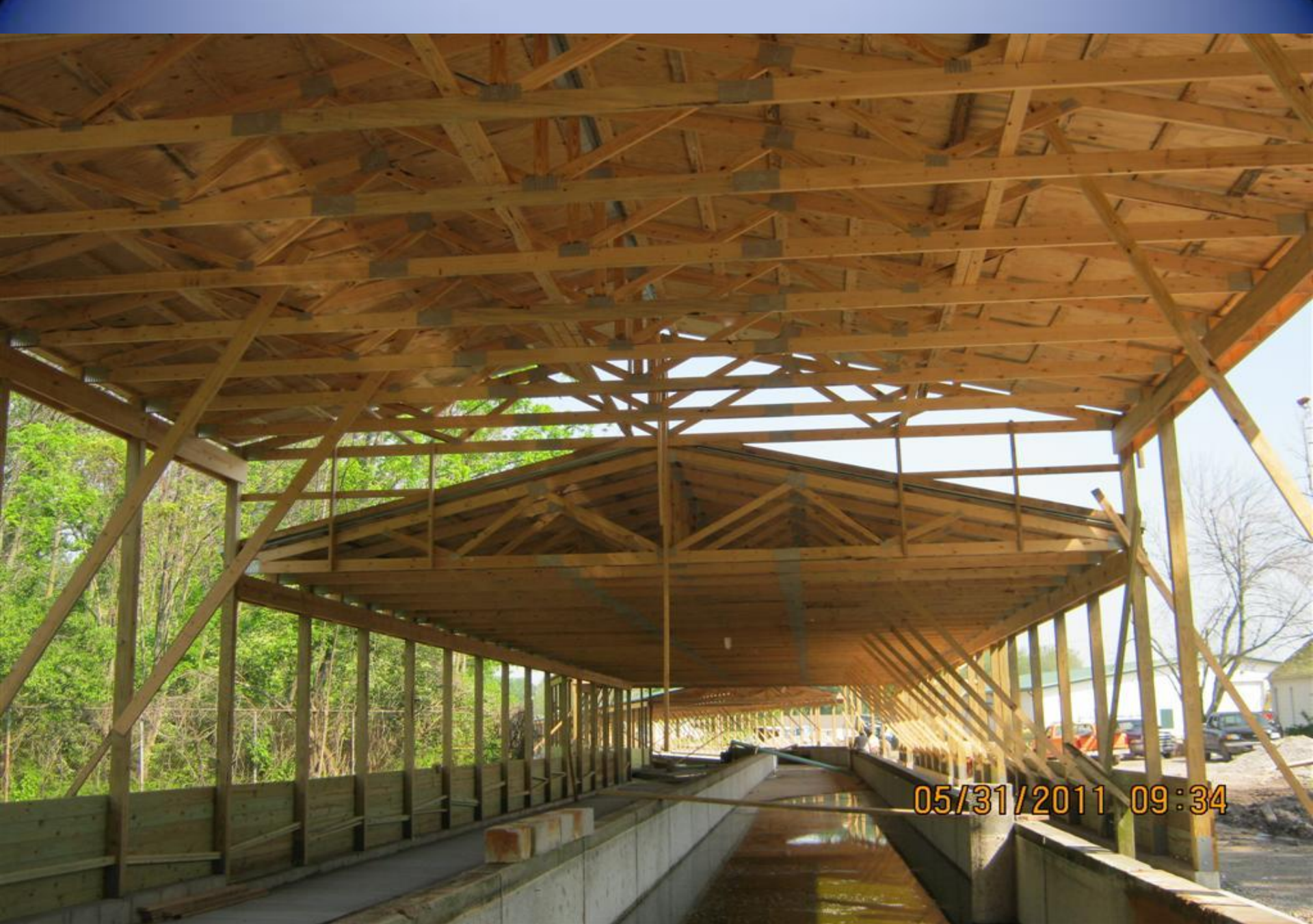
Construction continues on the Raceway Structure.
