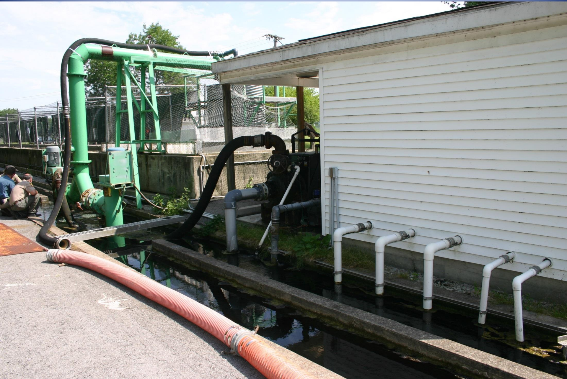
Original pump house and pumping facility
