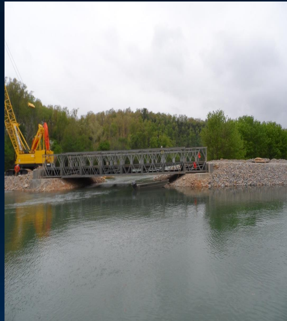
TEMPORARY BRIDGE PLACED
