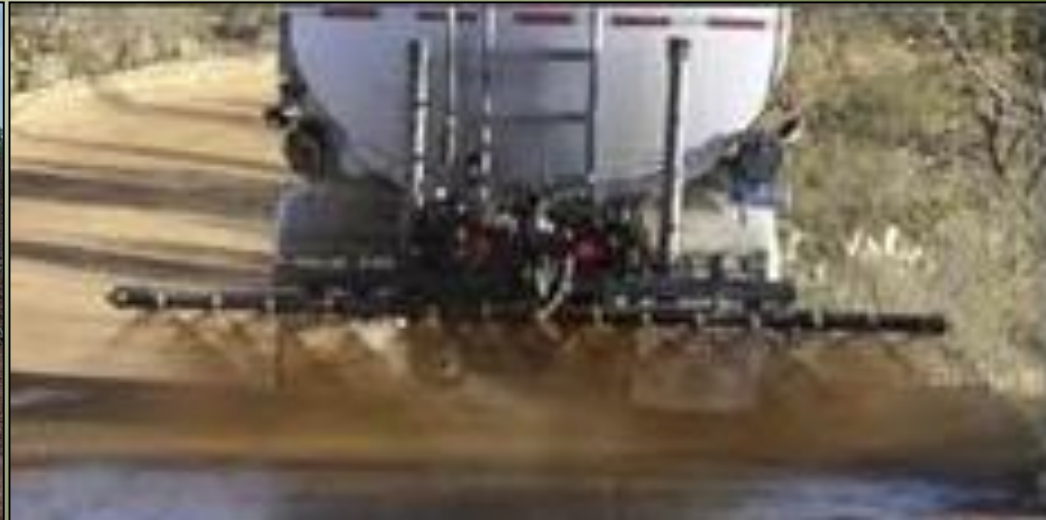
Lignosulfonate sprayed on road
