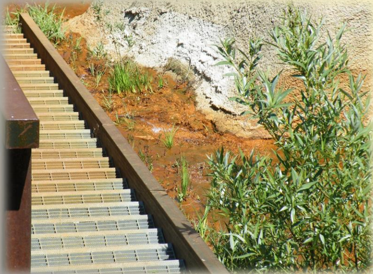
Seepage in Bay 5 has been reduced from 5 to 10 cfs to level that is difficult to measure. Stained rocks are the previous seepage path. Preconstruction are pictures on left. Post construction on right.
