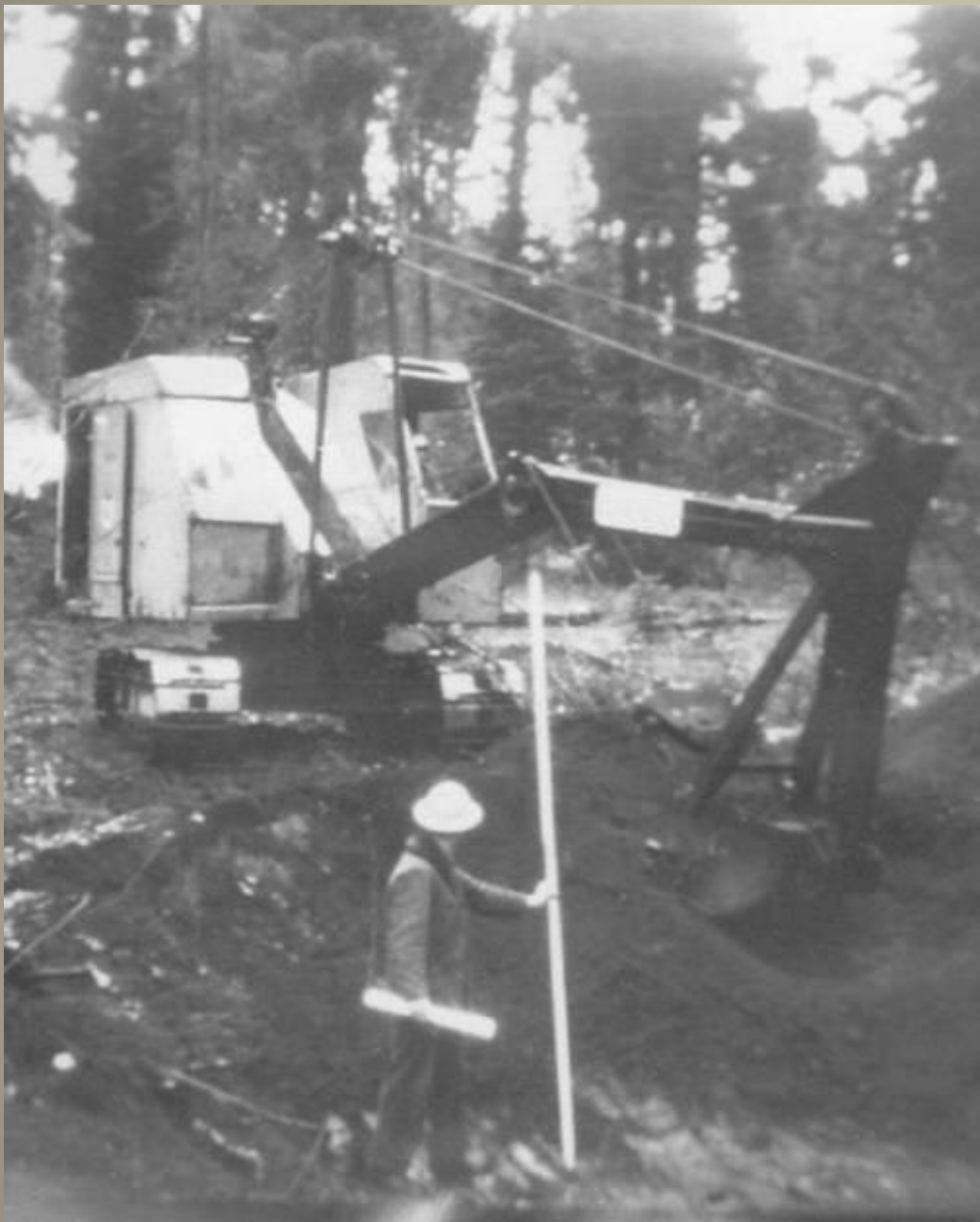
Start of excavation for the 1961 dam.
