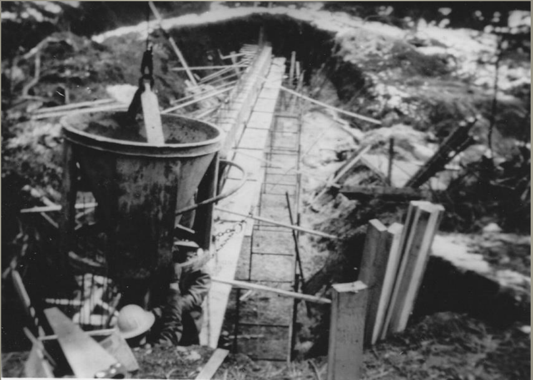
Pouring core wall for the 1961 dam.
