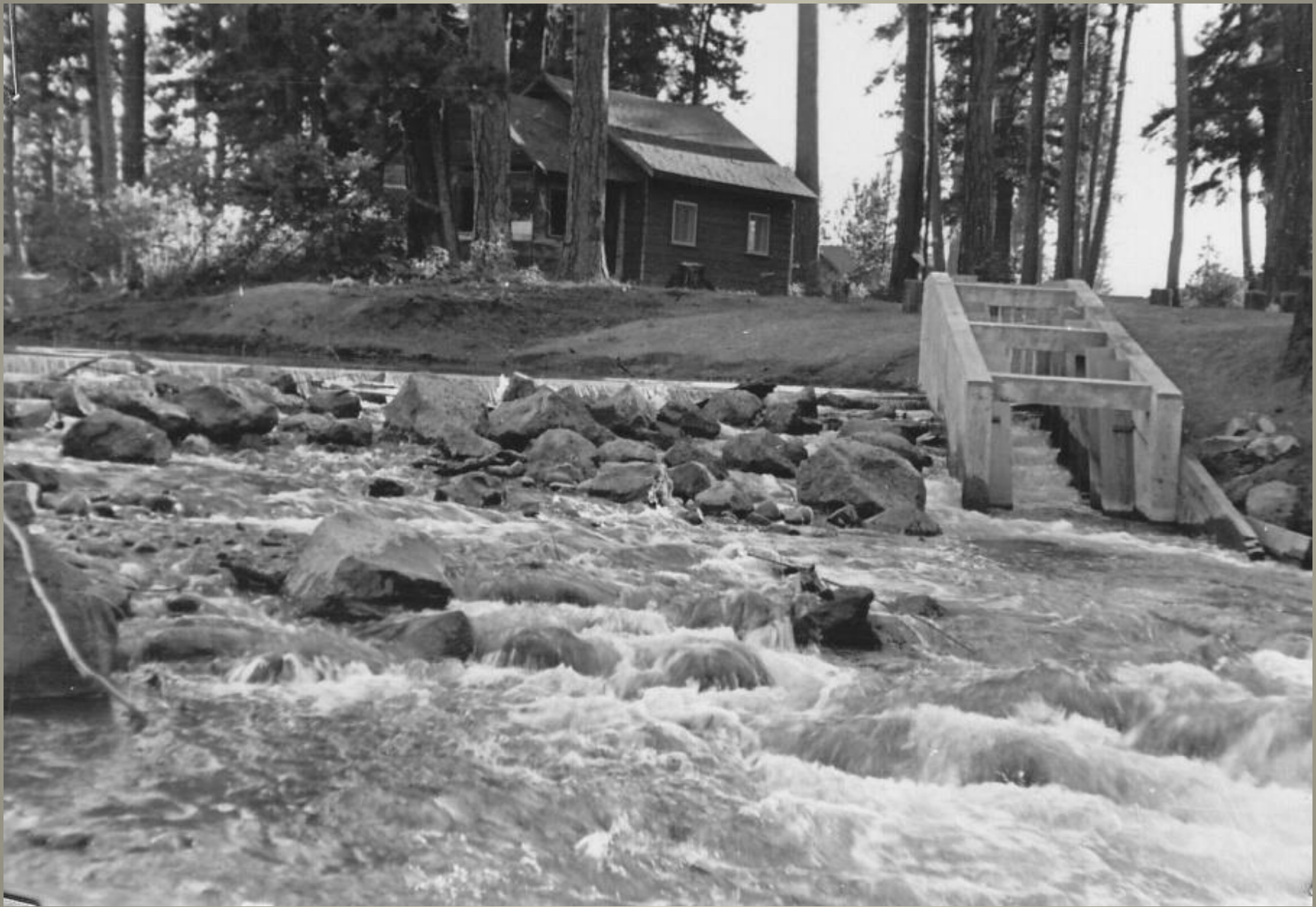
Completed 1961 dam with fish ladder.
