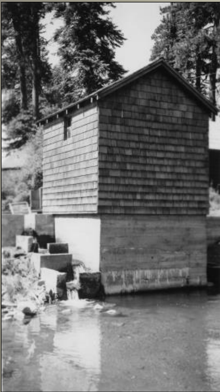
Powerhouse and fish ladder below dam at Suttle Lake outlet, 22 June 1942. Source: Pacific Northwest Stream Survey Photographic Collection, Oregon State University Archives, Corvallis, Oregon.
