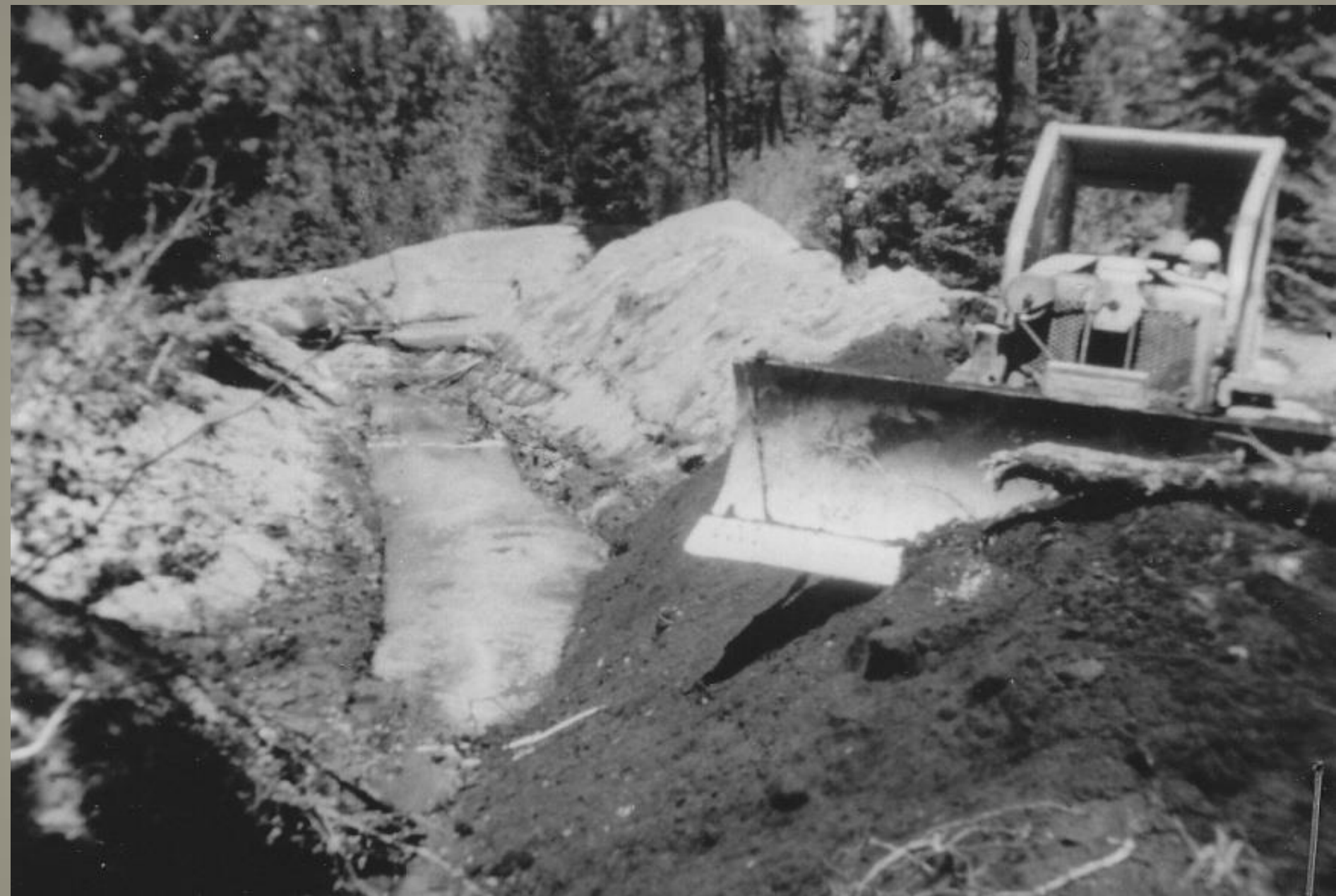
Filling in bypass channel for 1961 dam.
