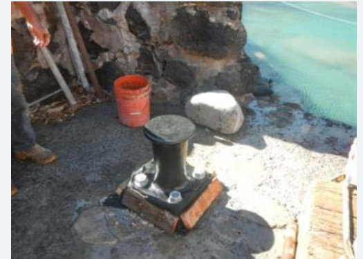
Installation of mooring bollard
