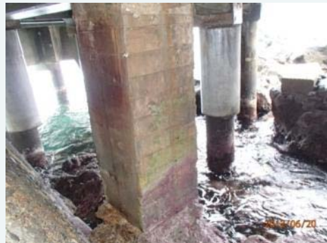
Concrete dock pile repairs
