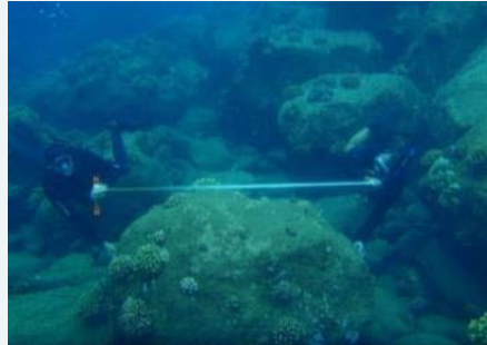
Displaced armor stone
