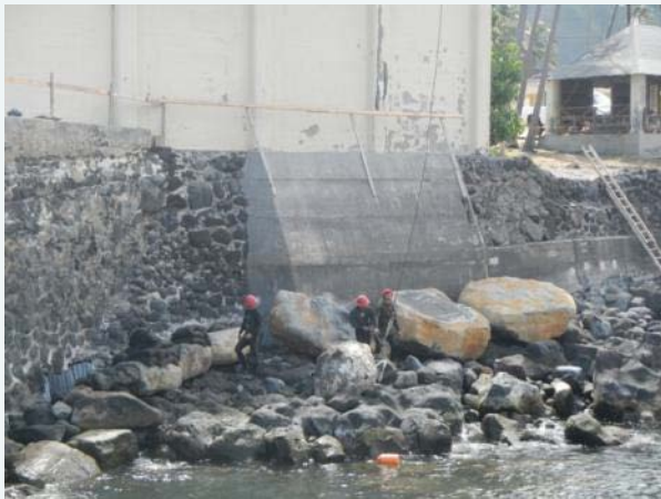
Armor stone placement
