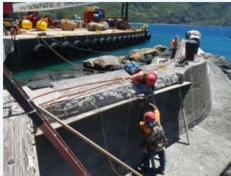
Breakwater spall demolition
