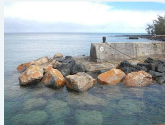
Armor stone at breakwater
