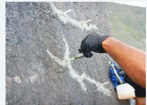
Crack sealing
