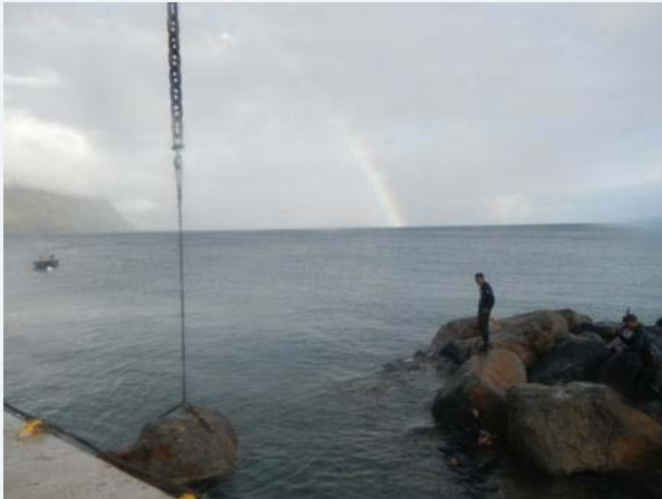
Armor stone relocation
