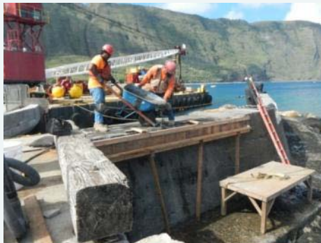
Placement of concrete at breakwater
