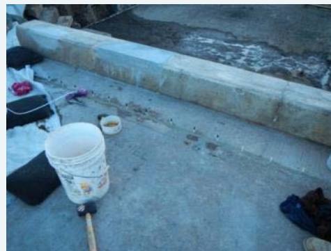
Crack sealing
