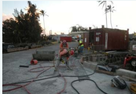
Demolition of slab
