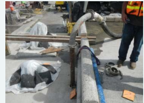
Stone bulkhead void filling
