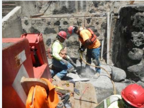
Drilling anchors
