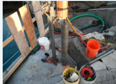
Concrete coring
