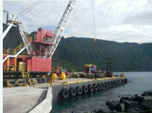
Armor stone relocation
