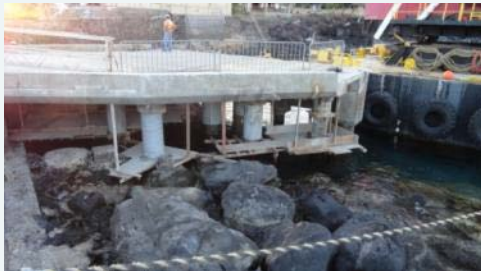
Concrete dock pile repairs
