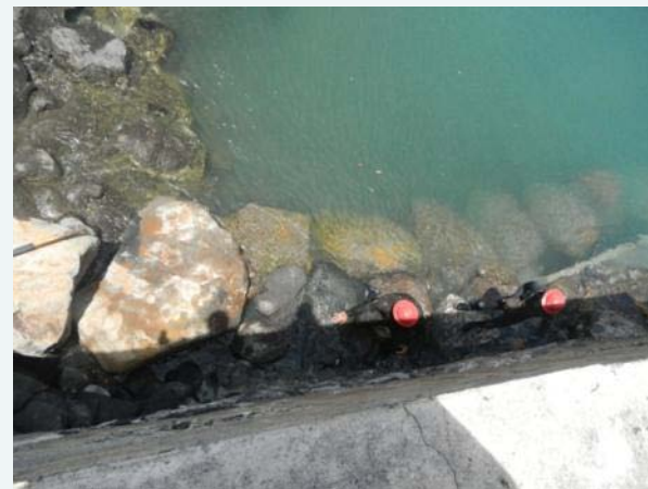
Armor stone placement
