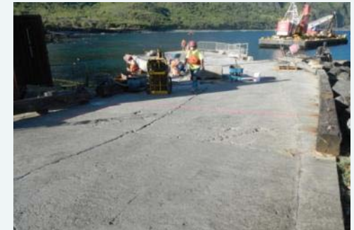
Demolition of top deck
