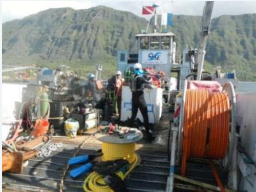
Mooring buoy installation
