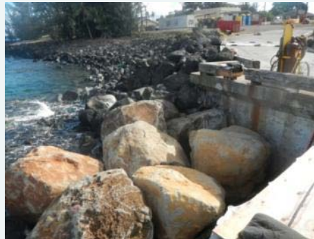
Armor stone placement
