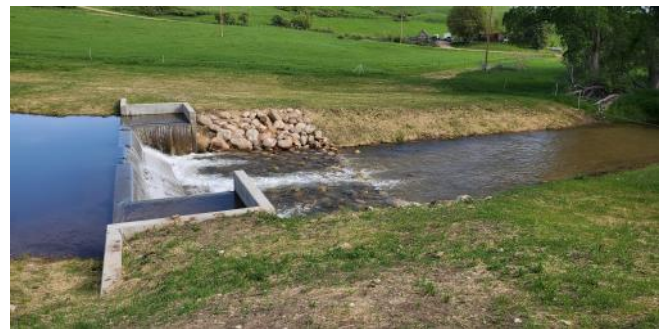
Fish barrier to limit brook trout passage in order to restore the yellowstone cutthroat population.
