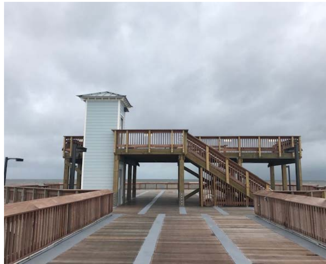
ADA LIFT TOWER AND STAIR FACADE
