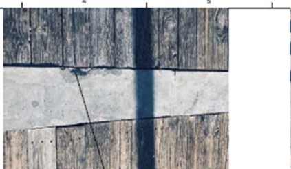
EXISTING CONCRETE DECKERS TO REMAIN. SCRAPE ALL LOOSE CONCRETE OFF. SAND BLAST, POWER WASH, CLEAN AND PREP FOR NEW CONCRETE COATING. TO DO: CLEAN, PATCH AND REPAIR ALL CONCRETE CRACKS AND UNBROKEN CORNERS. USE NEW CONCRETE WITH FINISH COATING. SHALL MATCH EXISTING TEXTURE AND BE P-RESISTANT FINISH. REFER TO STRUCTURAL FOR ADDITIONAL REFERENCE INFORMATION.
