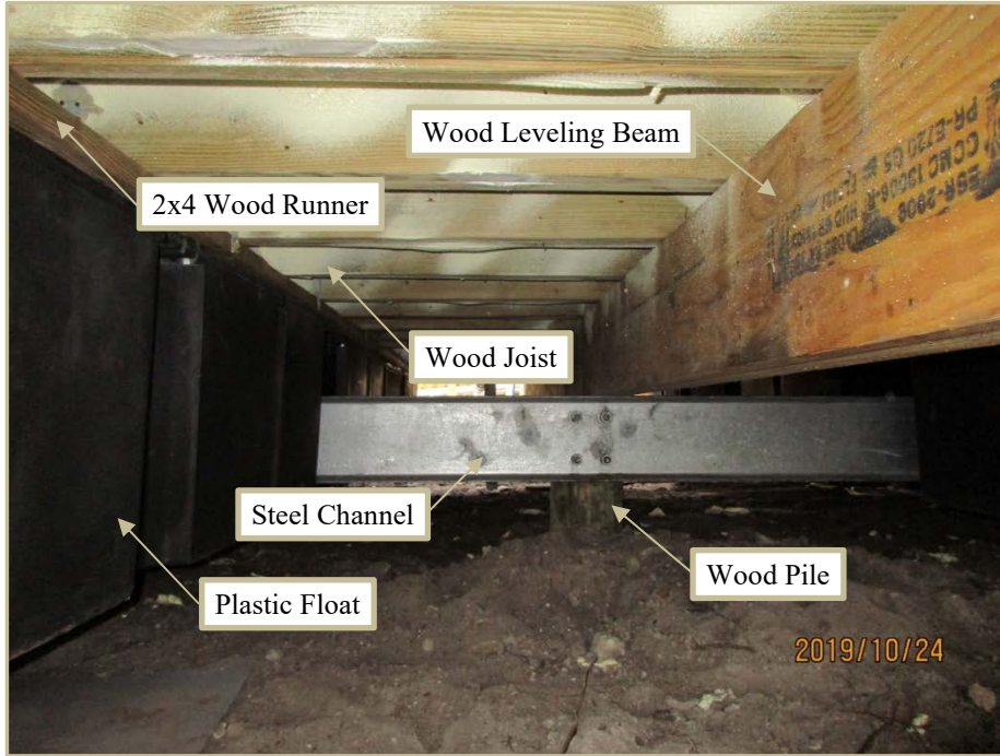
New cabin support structure and plastic floats
