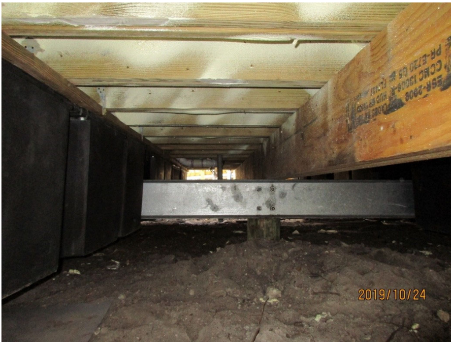
New cabin support structure and plastic floats.
