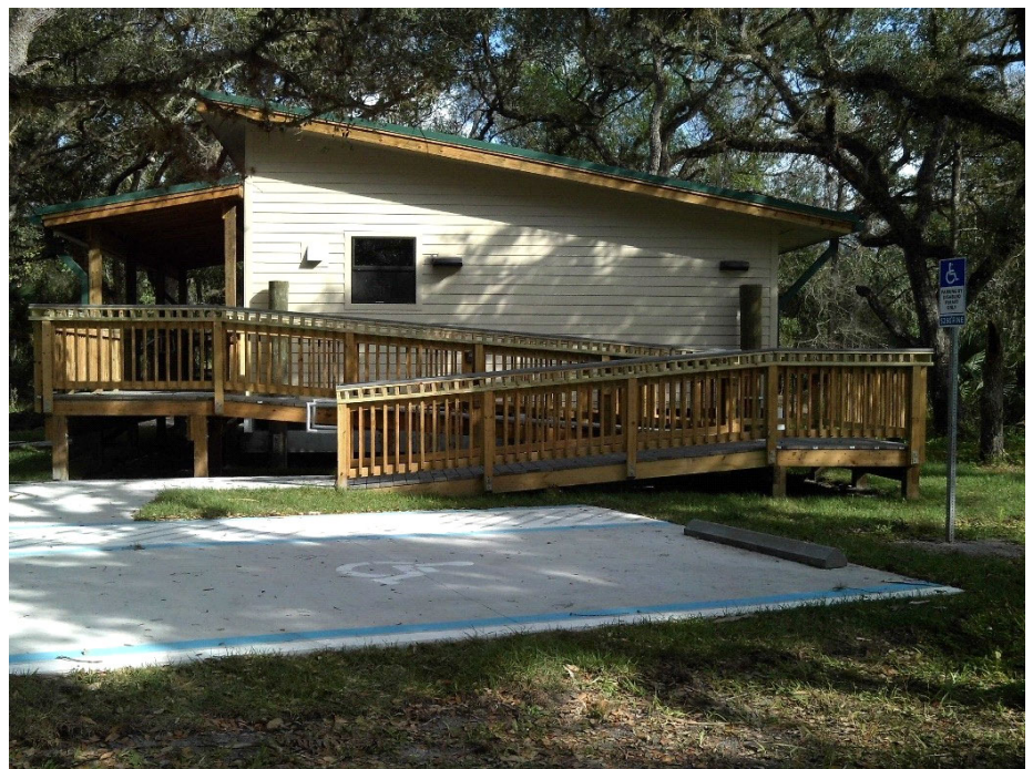
Stationary ADA access connected to front porch
