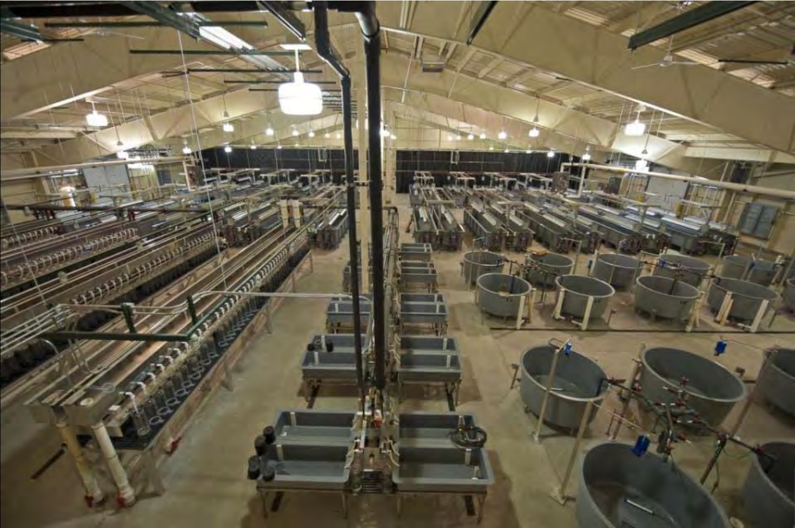
Interior of 30,000 SF Coolwater Production Building completed during Phase 2 of project
