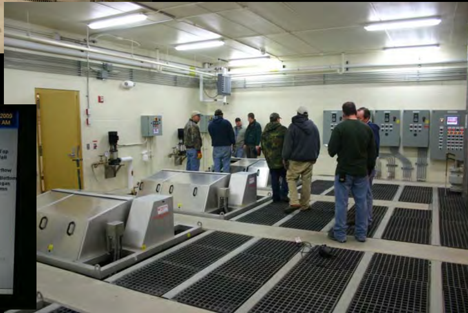
RAS Microscreens & Moving Bed Bioreactors
