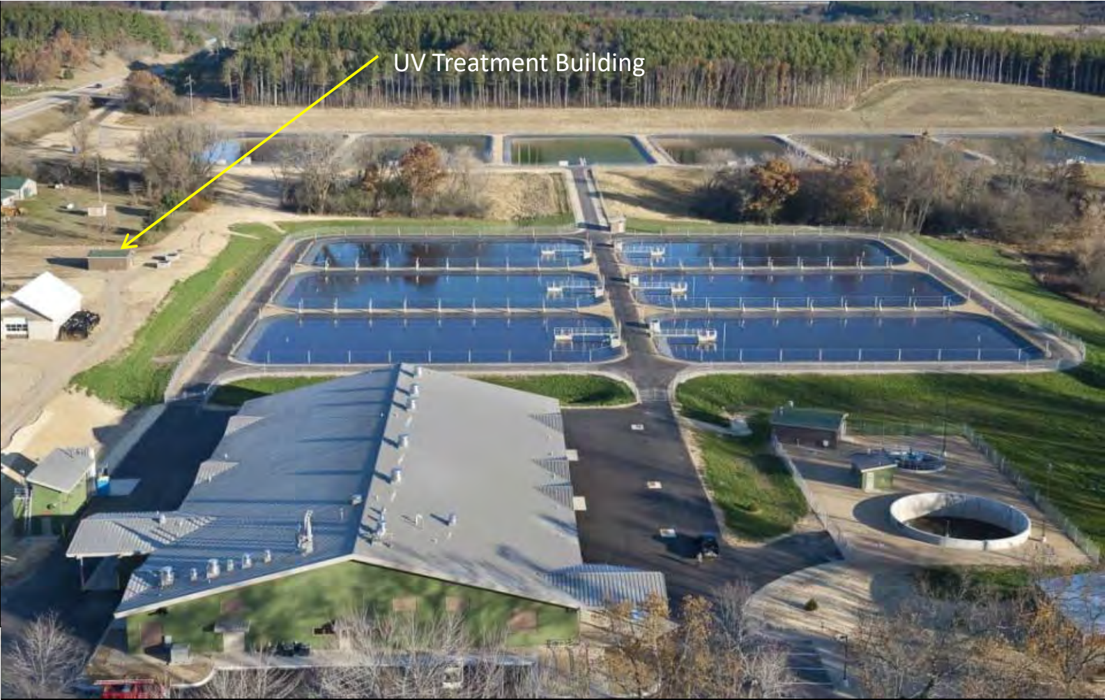
Coolwater hatchery completed in Phase 2 of project: Coolwater Production Building, sludge storage, clarifier, microscreening building, and pond complex
