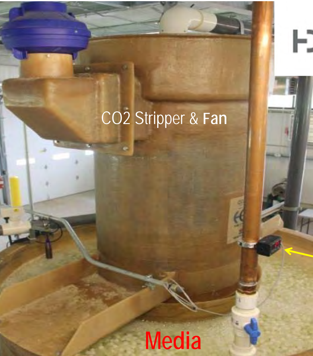
Moving Bed Biofilter & WaterTech Media Low Pressure Air Operated & Air Measurement
