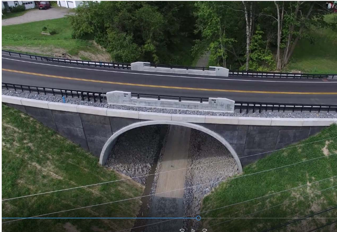
VT Route 2B Bridge Replacement, St. Johnsbury, VT
